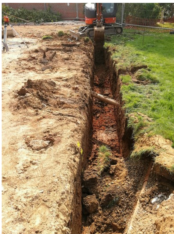
Photograph 4 Working shot trenching of main extension, view south
