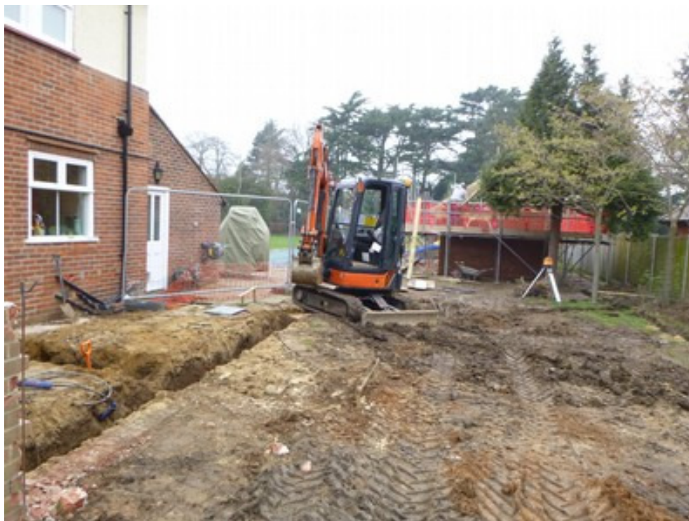
Photograph 3 Foundations of new garage with pool house, view west
