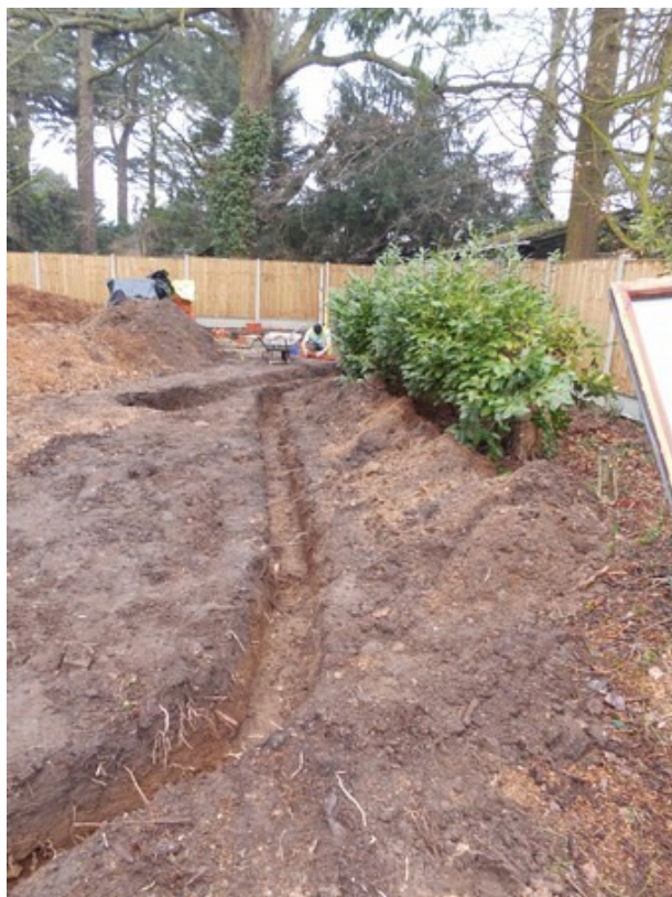
Photograph 1 Service trench and summer house, view west
