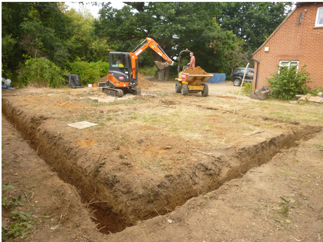
Photograph 1 Foundation trenches, looking northwest
