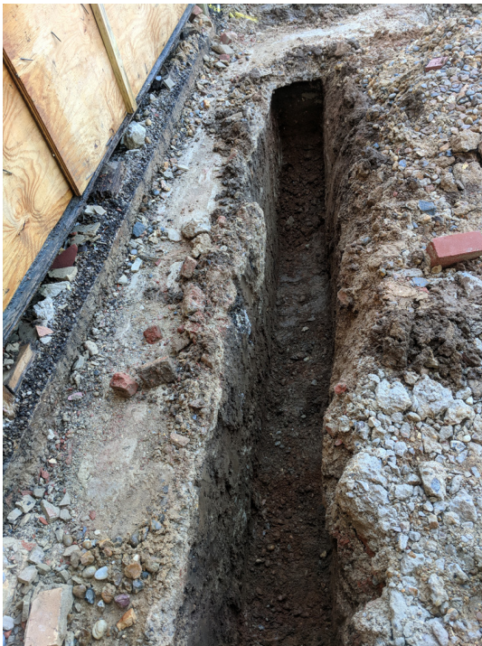
Photograph 1 Southern foundation trench, looking west
