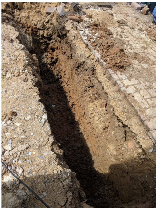
Photograph 2 Northern foundation trench, looking northwest
