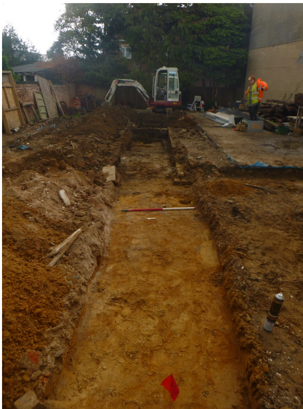
Photograph 1 First 4m of trenching, looking southeast
