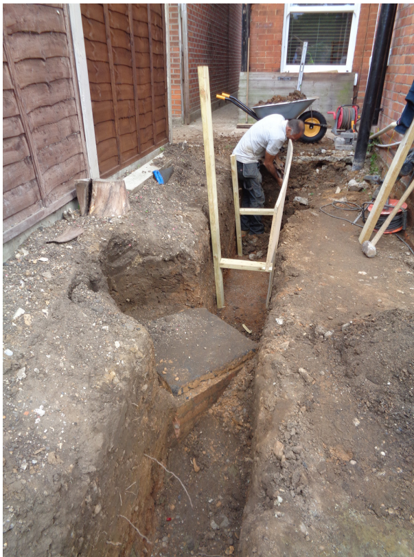
Photograph 2 Northwestern foundation trench, looking northeast
