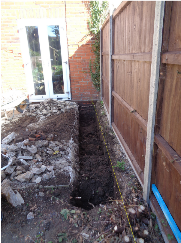
Photograph 1 Southeastern foundation trench, looking northeast
