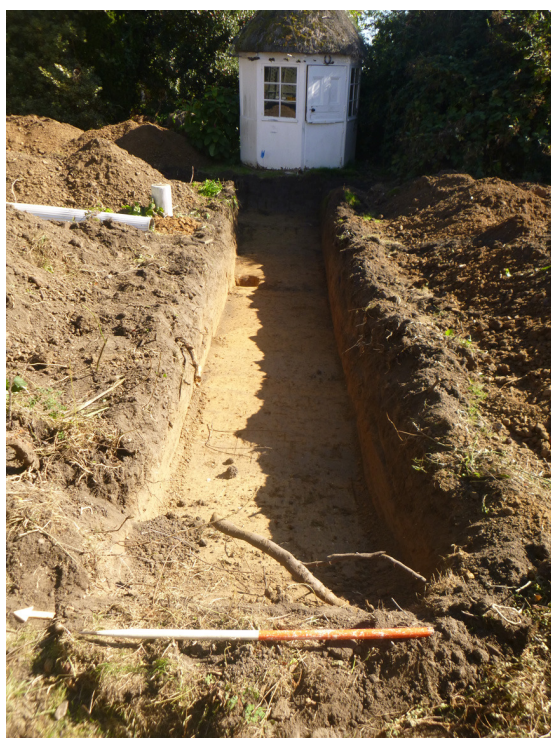
Photograph 2 Trench shot, looking east
