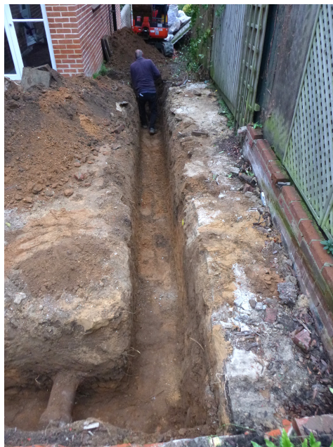
Photograph 1 Fully excavated trench
