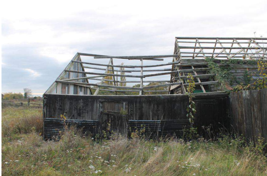
Photograph 25 North-east elevation of modern extension. Photograph taken facing south-west.
