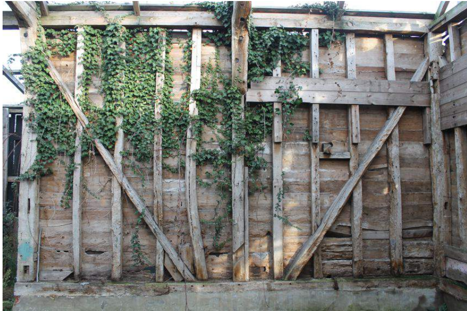
Photograph 6 East wall of Bays 1 and 2, showing primary-bracing. Photograph taken facing north-east.
