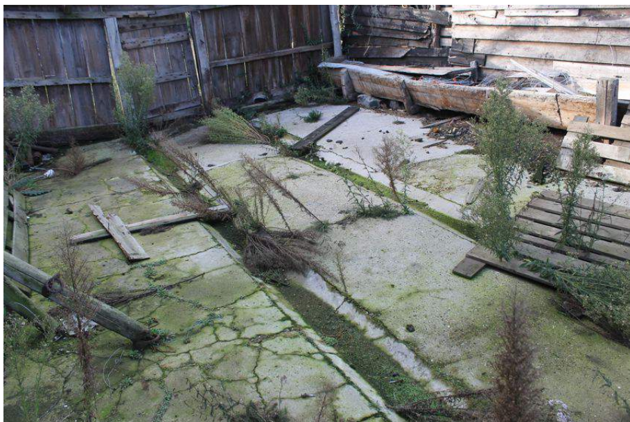
Photograph 26 Floor of extension, showing drainage channels. Photograph taken facing west.
