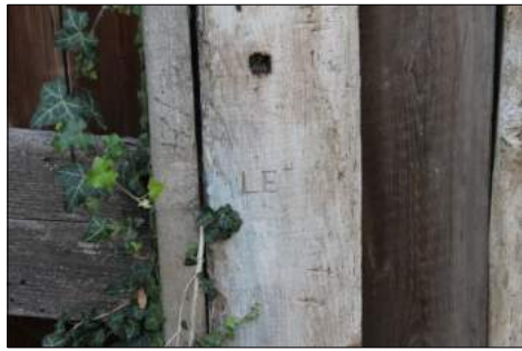
chiselled markings on interior of post
