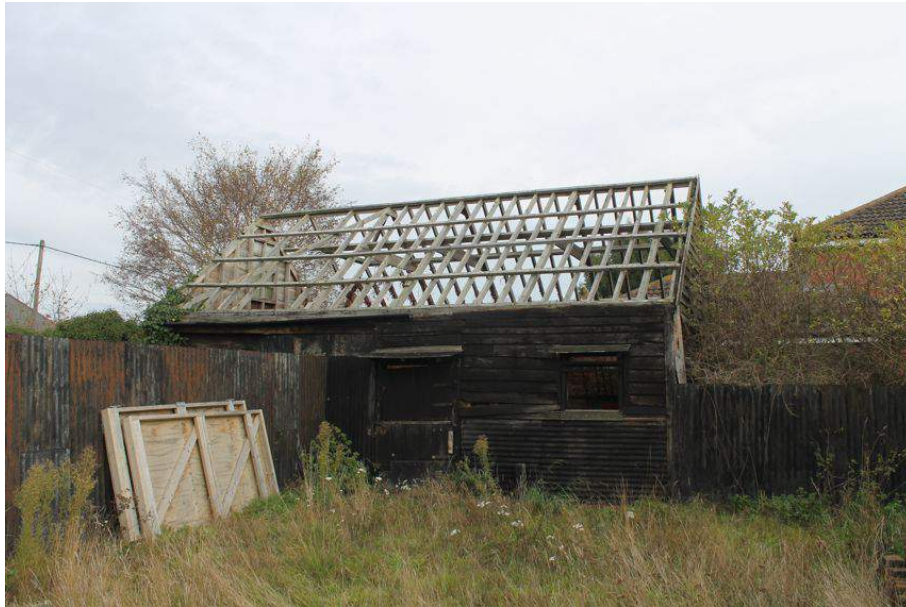
Photograph 28 South-west elevation of cow house. Photograph taken facing east.
