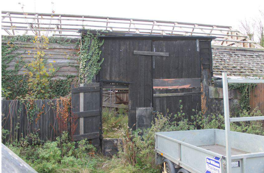
Photograph 2 Detail of the barn doors on north-east elevation of threshing barn's midstrey. Photograph taken facing west.
