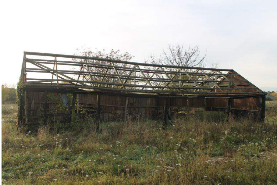
Photograph 45 North elevation of cart-lodge, with multiple entrances. Photograph taken facing south.
