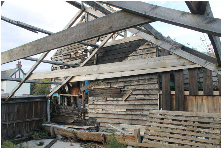
Photograph 27 Interior shot of extension, showing roof truss. Photograph taken facing north-west.
