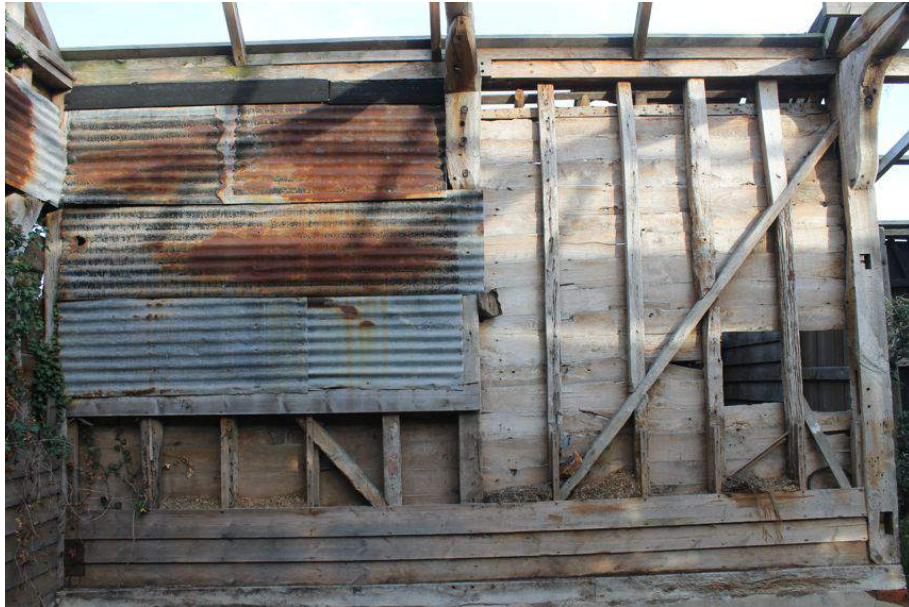
Photograph 14 East wall of Bays 4 and 5. Photograph taken facing north-east.
