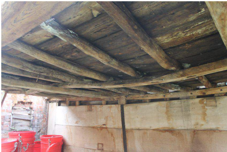
Photograph 38 Underside of first-floor, showing secondary binding-beam. Photograph taken facing east.
