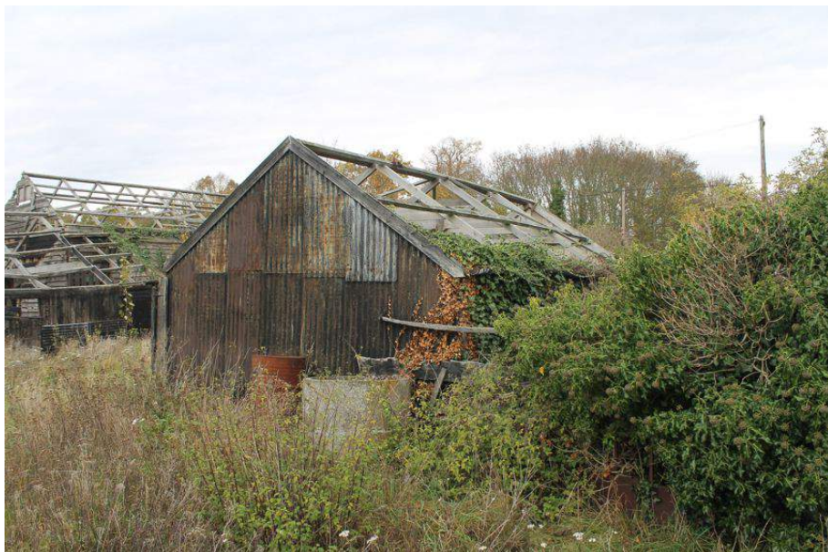
Photograph 41 South-east and north-east elevations of stables. Photograph taken facing north-west.
