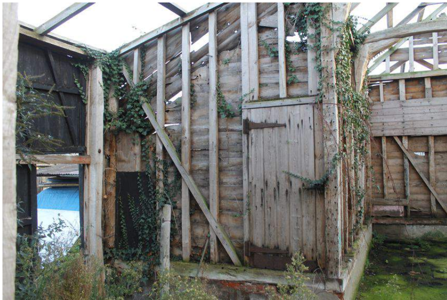
Photograph 19 South wall of the barn's midstrey. Photograph taken facing south-east.
