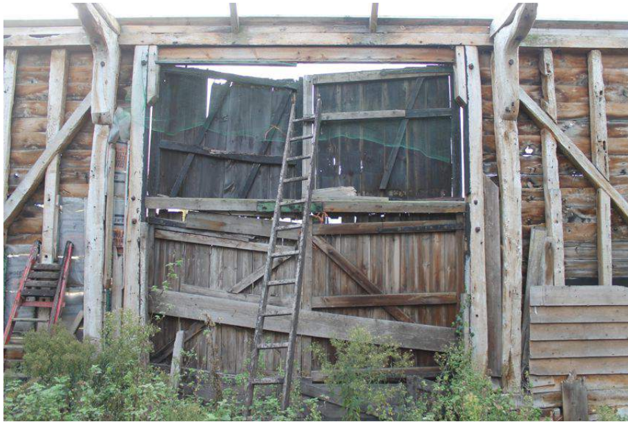
Photograph 12 Detail of barn doors in Bay 3. Photograph taken facing south-west.
