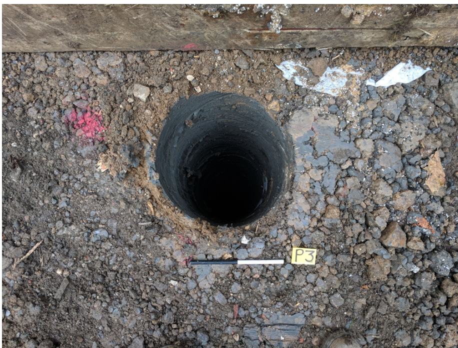
Photograph 3 Pile-hole, looking W
