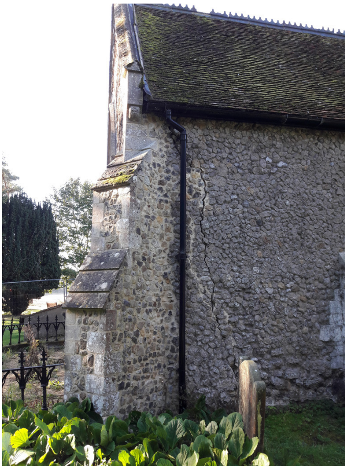
Photograph 1 Crack through the chancel wall, looking S
