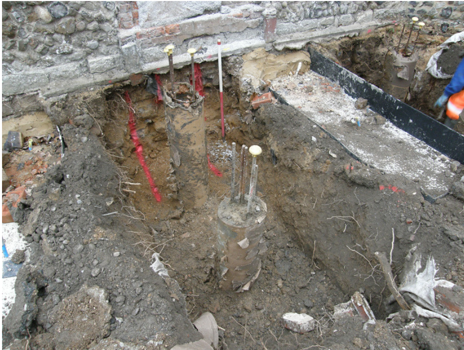
Photograph 4 Excavation of the ground-beams around the pile caps, looking NW
