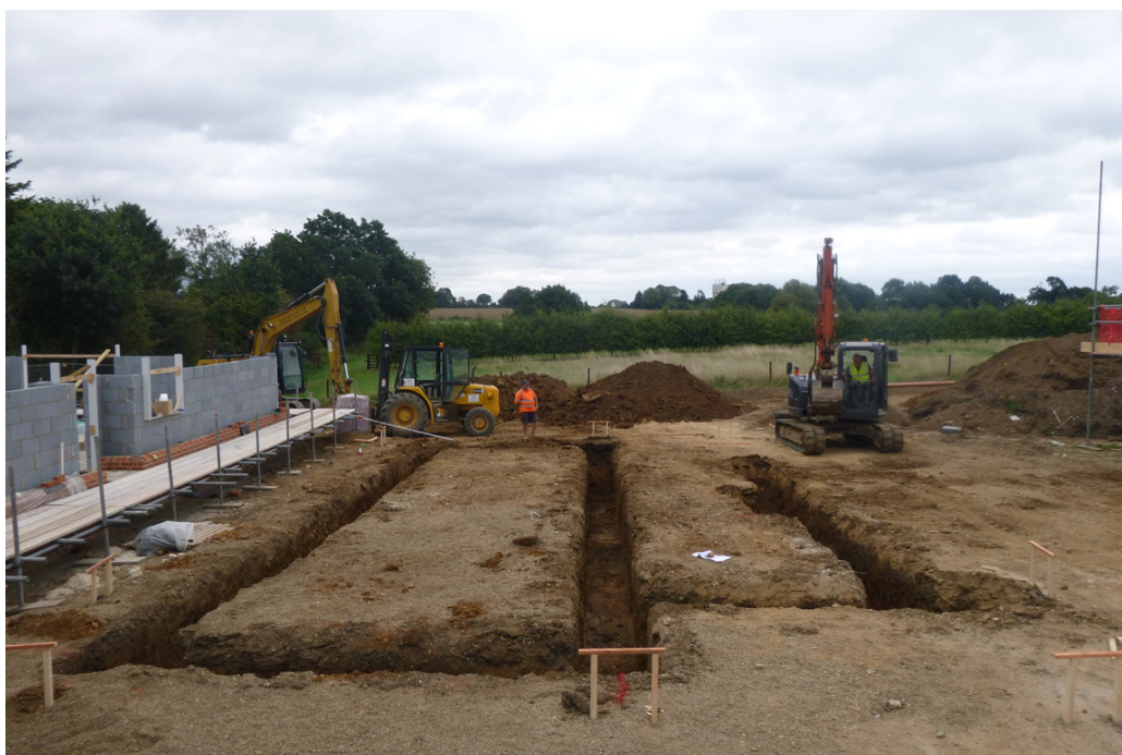
Photograph 2 Foundation trenches, looking east
