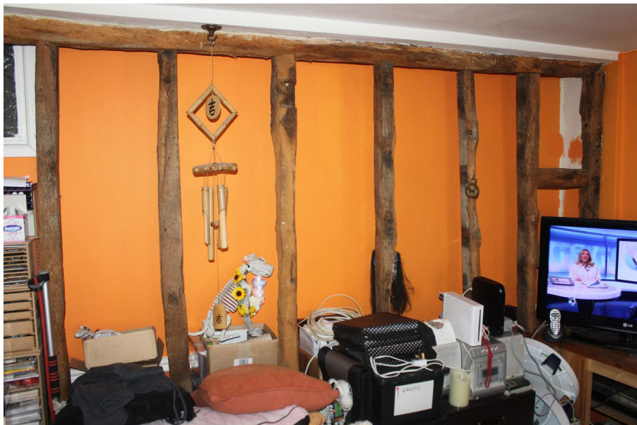
Photograph 19 Imitation timber wall in northern-room of ground-floor. Photograph taken facing south-west.
