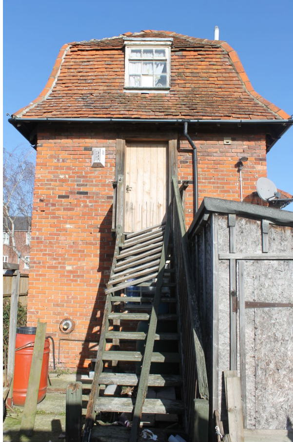
Photograph 11 Southern elevation of extension, showing staircase up to first-floor door. Photograph taken facing north.
