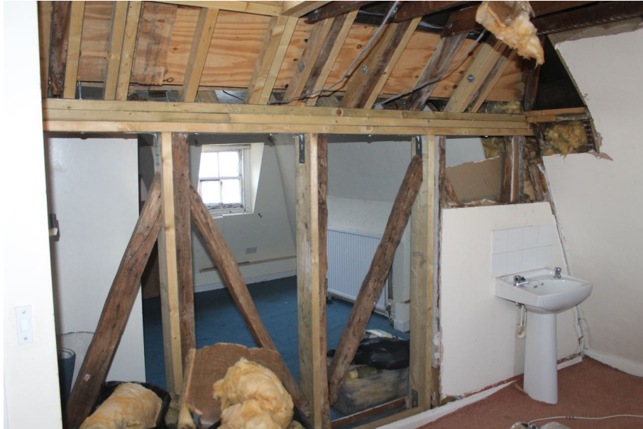
Photograph 26 Timber wall between north-west and south-west room in main range on second-floor. Mixture of modern machine-cut and historic hand-sawn timber visible. Photograph taken facing south-west.
