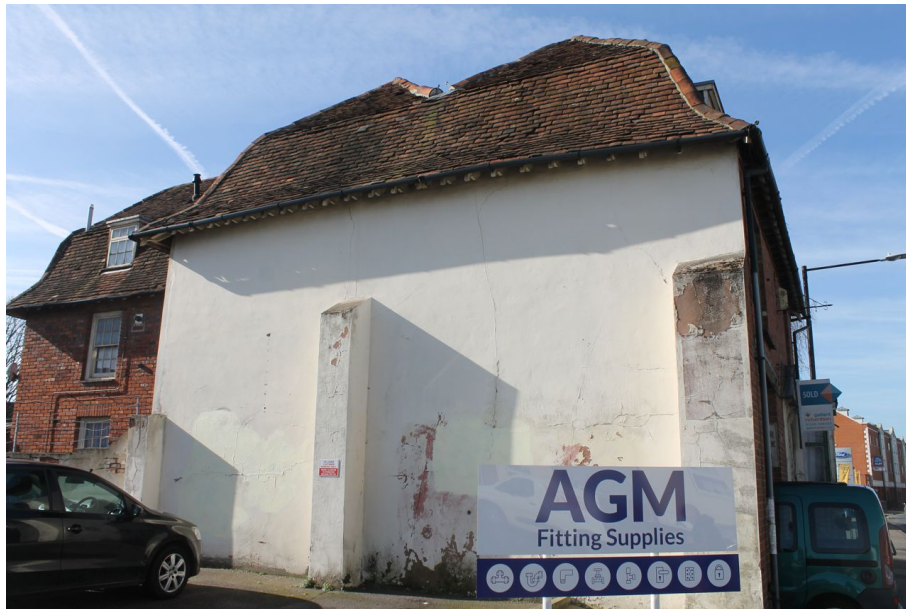
Photograph 7 East elevation of 79 Magdalen Street. Photograph taken facing south-west.
