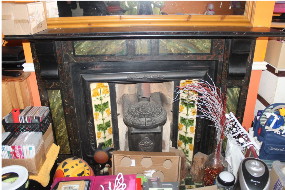
Photograph 18 Tiled fireplace surround in northern room of ground-floor. Wood burner in centre a modern insertion. Photograph taken facing west.
