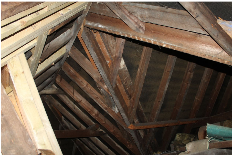
Photograph 27 Roof structure, showing extension's roof to right attaching to main ranges roof. Photograph taken facing east.
