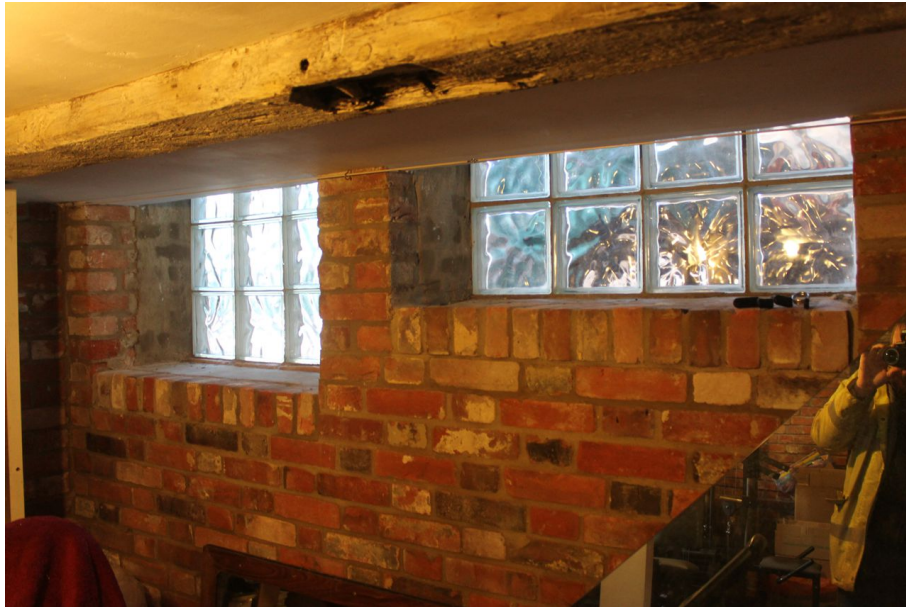
Photograph 14 Hammered-glass windows on east side of cellar, looking out onto passageway. Photograph taken facing north-east.
