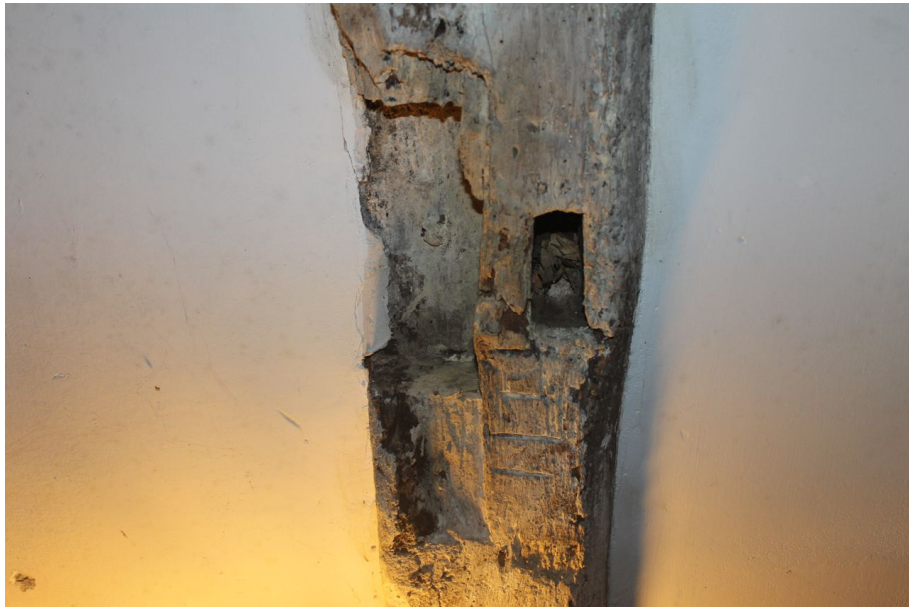
Photograph 17 Detail of empty mortise and carpenter's mark "IIII" on underside of joist in cellar.
