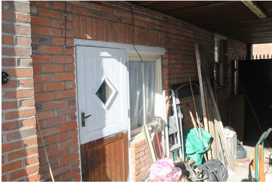
Photograph 9 Western wall of passageway on ground-floor of 79 Magdalen Street, showing rebuilt wall. Photograph taken facing north-west.
