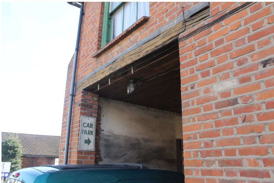
Photograph 6 Entrance into passage leading to rear of building on northern elevation. Substantial timber lintel visible. Photograph taken facing south-east.
