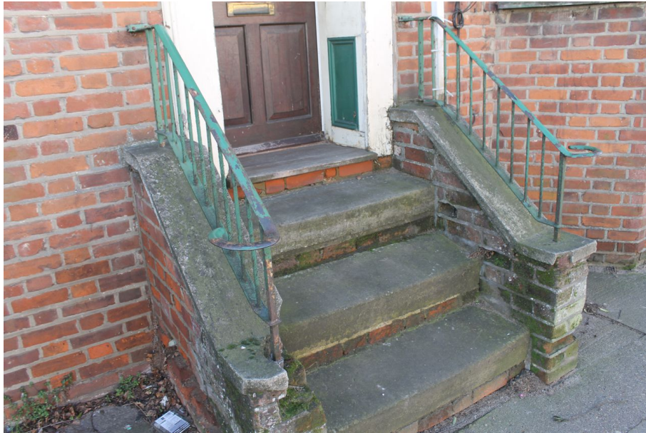
Photograph 5 Detail of steps up to front door on northern elevation of 79 Magdalen Street. Photograph taken facing south-west.
