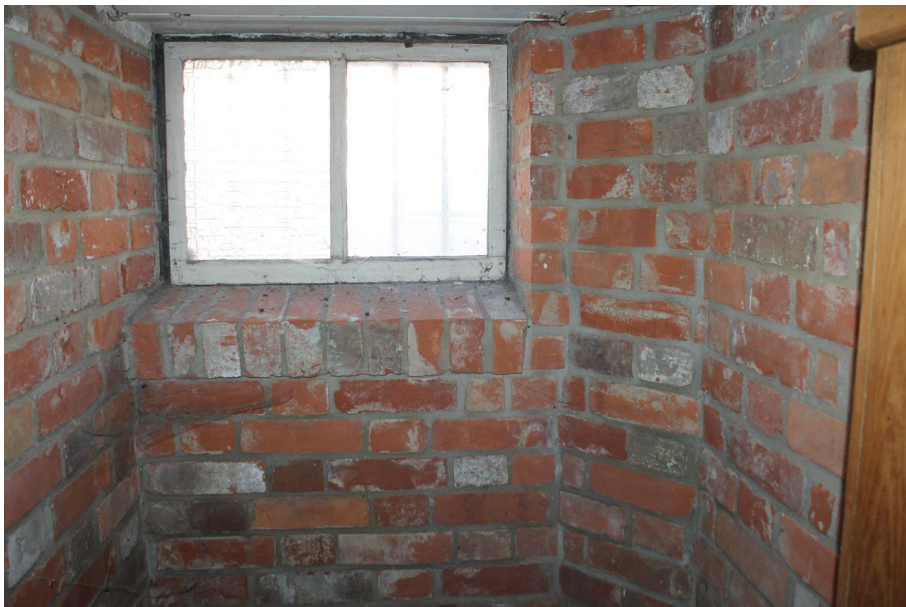
Photograph 15 Fixed window in cellar below bay window on ground-floor. Rebuilt brickwork around. Photograph taken facing north.
