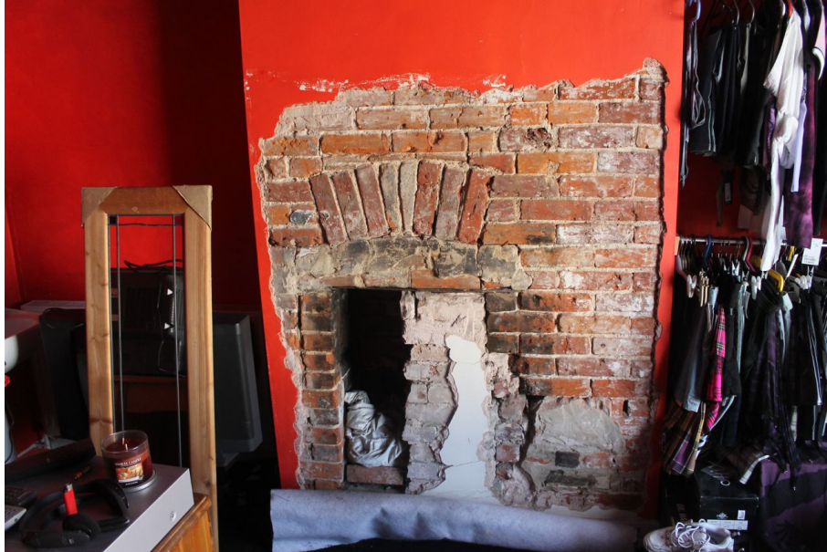
Photograph 22 Blocked then partially reopened northern fireplace on first-floor. Photograph taken facing west.
