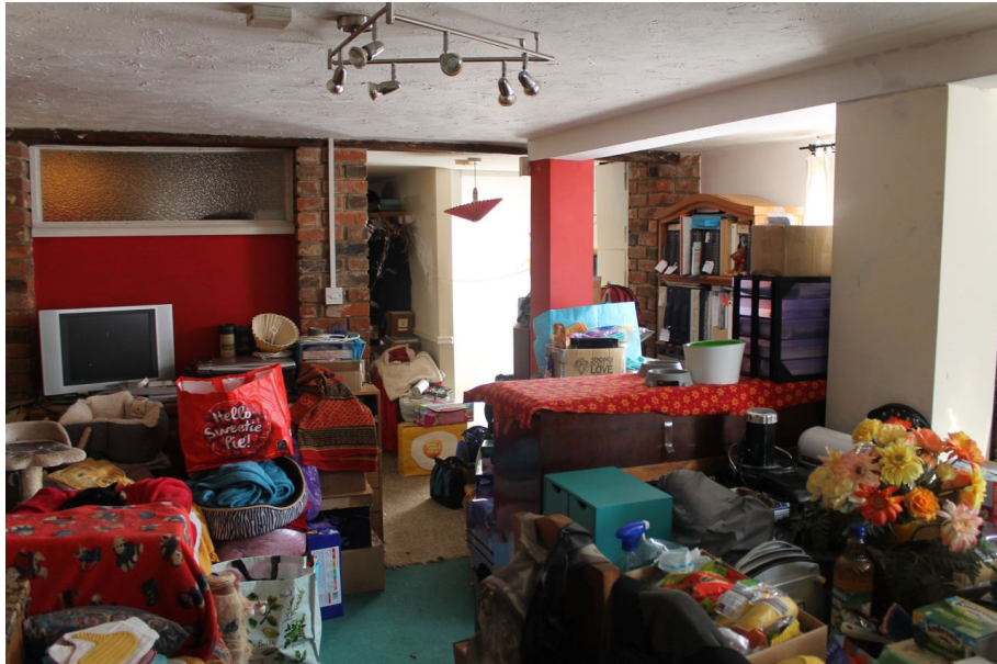
Photograph 20 Ground-floor of extension, showing brick pillars supporting upper floors of main range. Photograph taken facing north.
