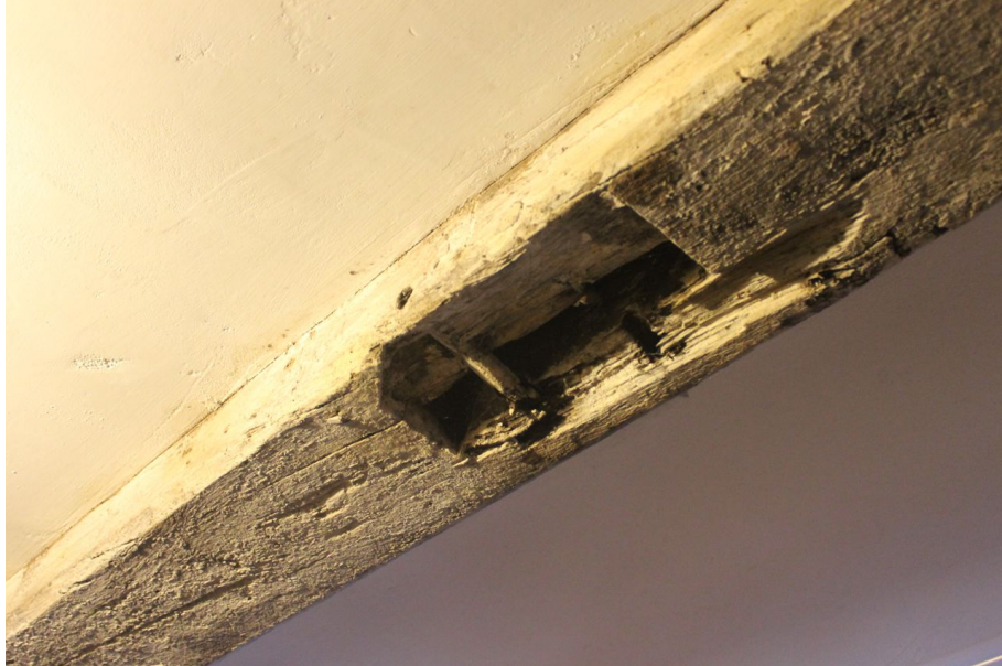
Photograph 16 Detail of empty mortise on joist in cellar. Photograph taken facing north-east.
