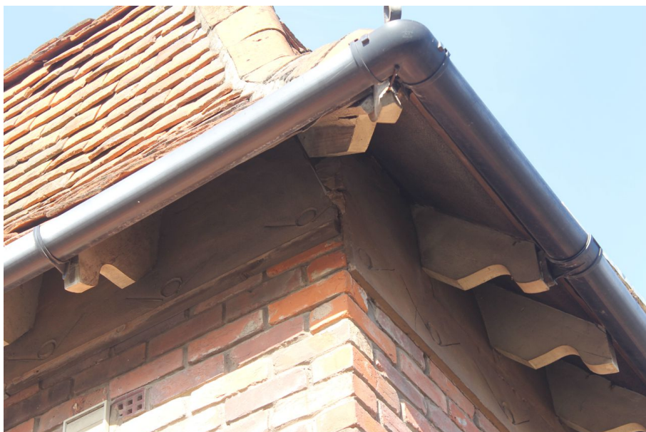
Photograph 2 Detail of cornice around entire building. Chamfered rafter-ends and incised cement shown.
