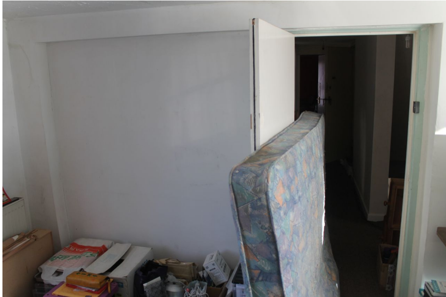
Photograph 24 View from extension showing entrance into main range on first-floor, alongside possible blocked entrance or window. Photograph taken facing north.
