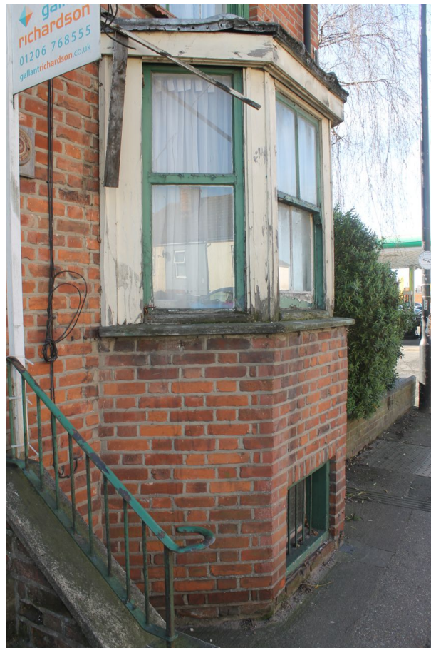
Photograph 4 Bay window on northern elevation of 79 Magdalen Street. Photograph taken facing south-west.
