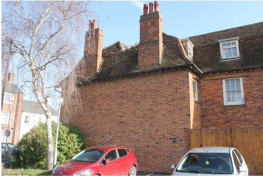
Photograph 3 Western elevation of 79 Magdalen Street. Two chimney-stacks visible on main range. Photograph taken facing north-east.
