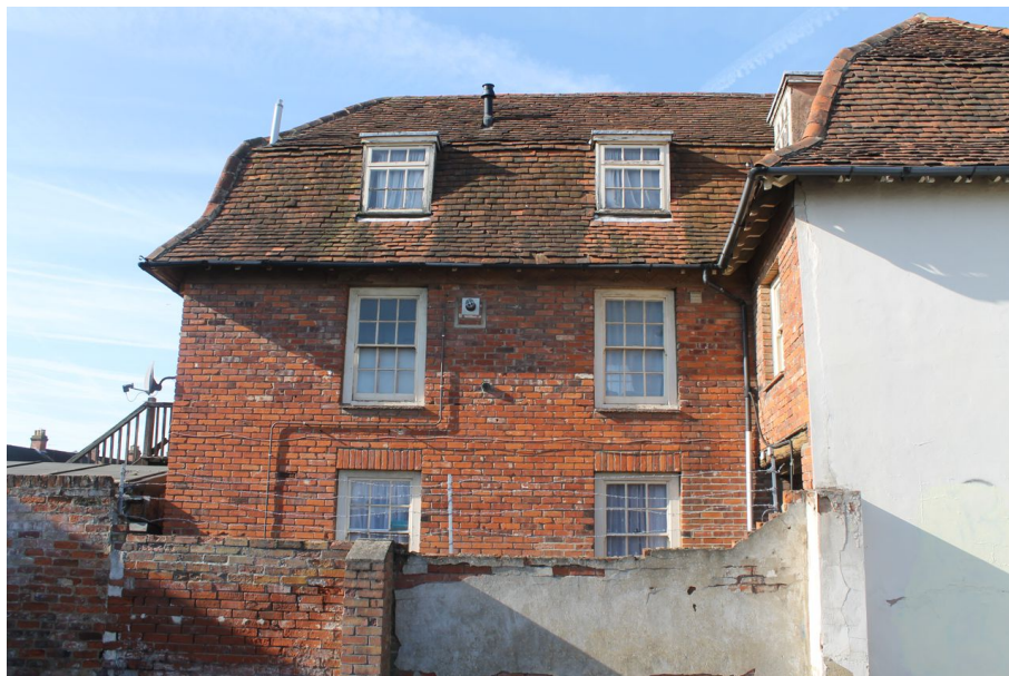
Photograph 8 East elevation of extension. Photograph taken facing west.
