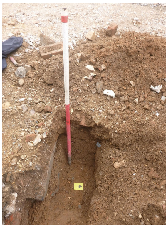
Photograph 2 A service trench at the eastern edge of the development area, looking west
