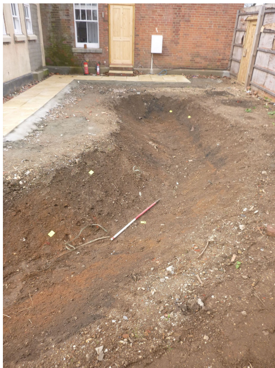
Photograph 4 Modern ?pit F1 (beneath the ranging rod) and the backfilled excavation area (the dark material in the northern face of the face swale), looking west
