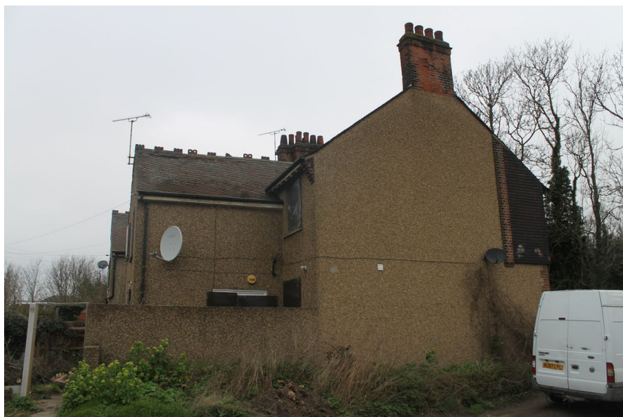
Photograph 5 South-east elevation of No 12. Photograph taken facing north-west.
