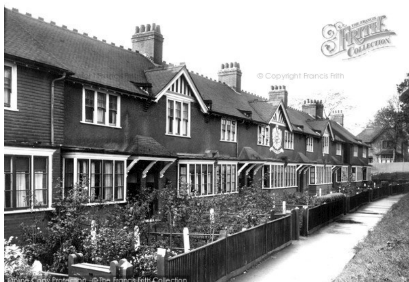
Photograph 3 North elevation of Botany Cottages. No 10 and 11 visible to left of frame. Taken from www.francisfrith.com .
