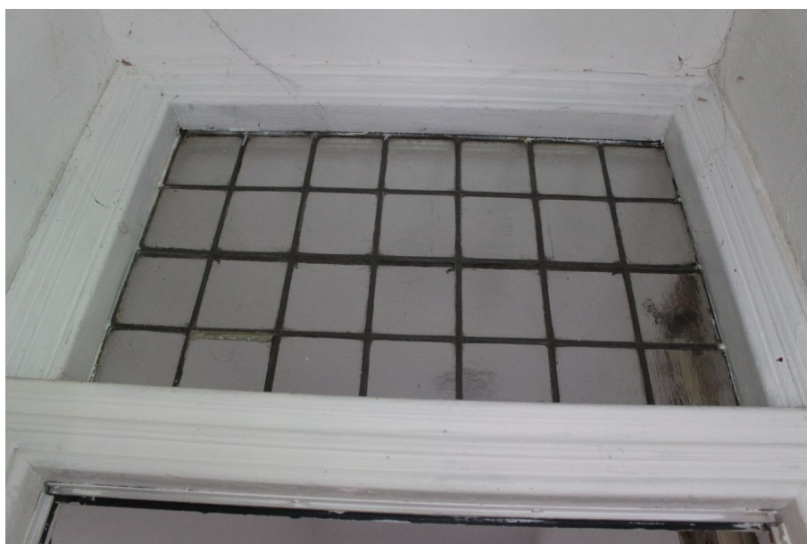
Photograph 10 Detail of original leaded light in entranceway of No 10 on ground-floor. Photograph taken facing north-east.
