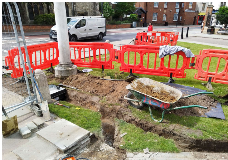
Photograph 2 Service trenching – looking southwest
