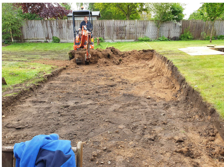
Photograph 1 Working shot showing stripped area.
