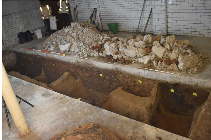
Photograph 1 TP1 west-facing sx oblique view – looking northeast
