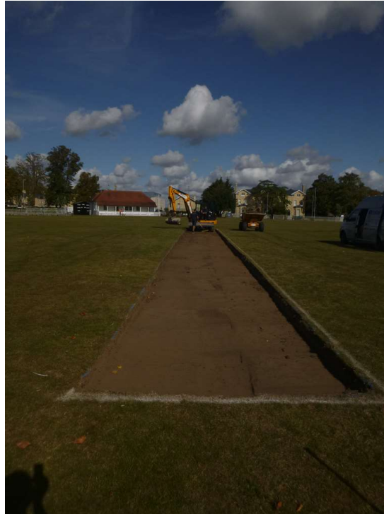
Photograph 1 Stripped area – looking north northwest
