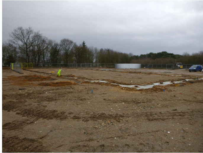
Photograph 5 Site shot after concreting – looking northeast
