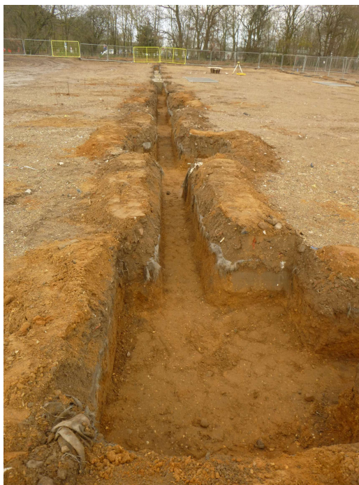
Photograph 3 Foundation pads, west side of building – looking north
