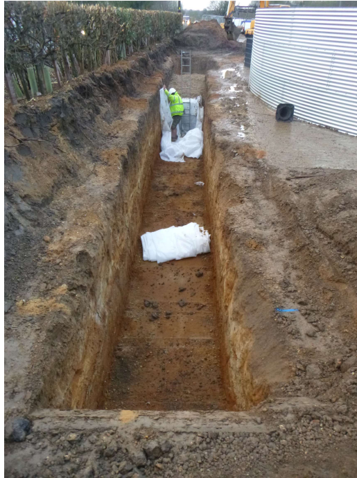
Photograph 7 Drainage trench east of water tank 1 – looking south
