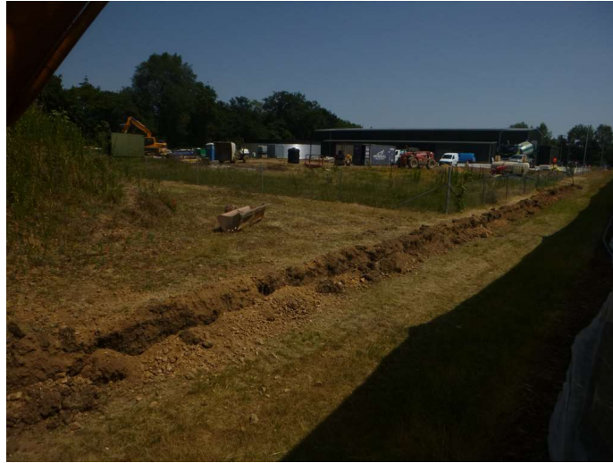
Photograph 10 Drainage trench to west of development site – looking northeast
