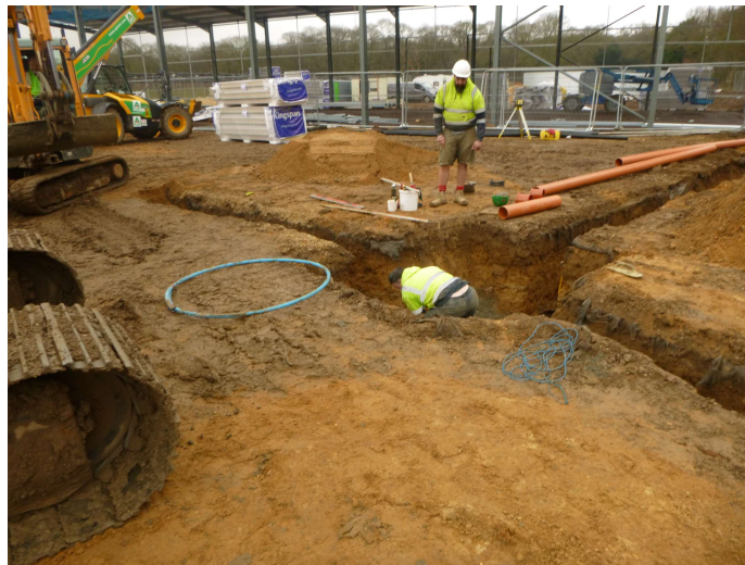
Photograph 6 Drainage trench east of new building – looking west
