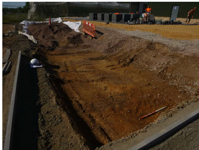
Photograph 8 Strip for drainage trench under grasscrete parking – looking south
