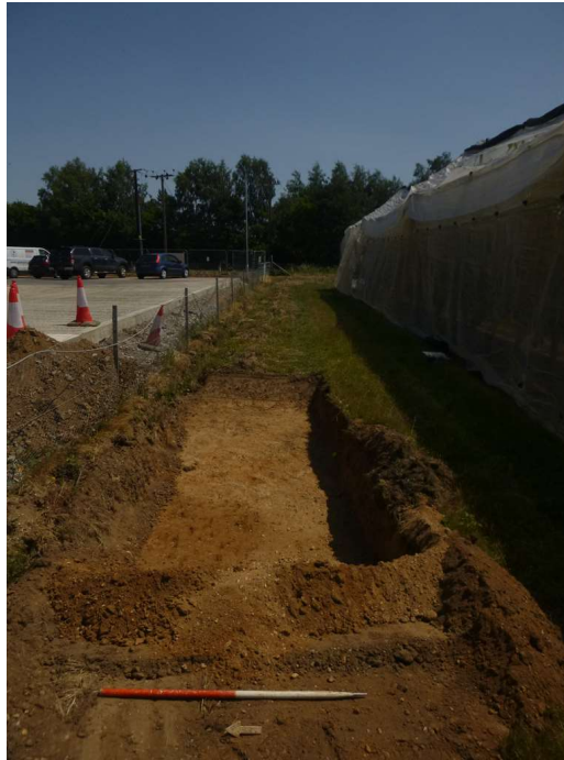
Photograph 9 Groundworks for waste water tank from butchery area – looking east
