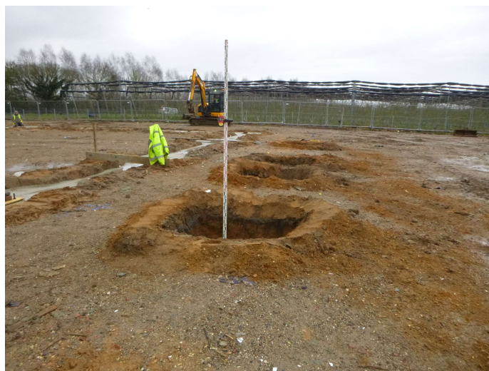
Photograph 4 Satellite pads, west side of building – looking south
