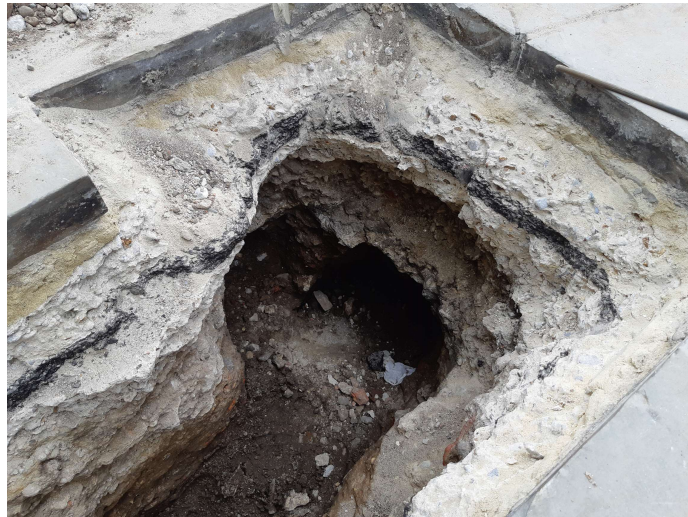
Photograph 1 Contractors' pit – looking southwest
