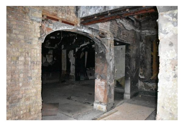
**Plate 26** Inserted arch leading into bar with removed wall to right, both supported by metal beams - view west.
