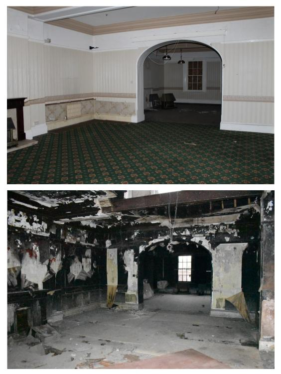
Plate 12 The 1904 bar converted from the quarters for Officers Nos.2 and 3, with the extension through the archway and the inserted fireplaces on the left-hand walls – view west. Photo from November 2013 above, photo from December 2019 below.
