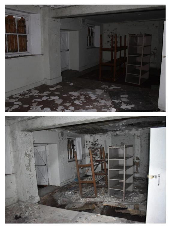
Plate 22 Rooms 39 and 38, the former kitchen and mess manager's room, with the dividing wall removed and a doorway inserted through one of the windows of the mess manager's room – view south. Photo from November 2013 above, photo from December 2019 below.
