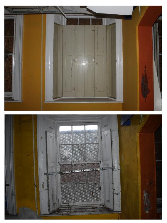
Plate 7 Example of the sash windows with recessed wooden shutters in the ground floor rooms of the 1874-5 building - view south-east. Photo from November 2013 above, photo from December 2019 below.
