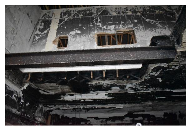
**Plate 25** Metal beam that would have supported the floor of room 22 prior to the fire. Herringbone strutting visible behind - view south-east.
