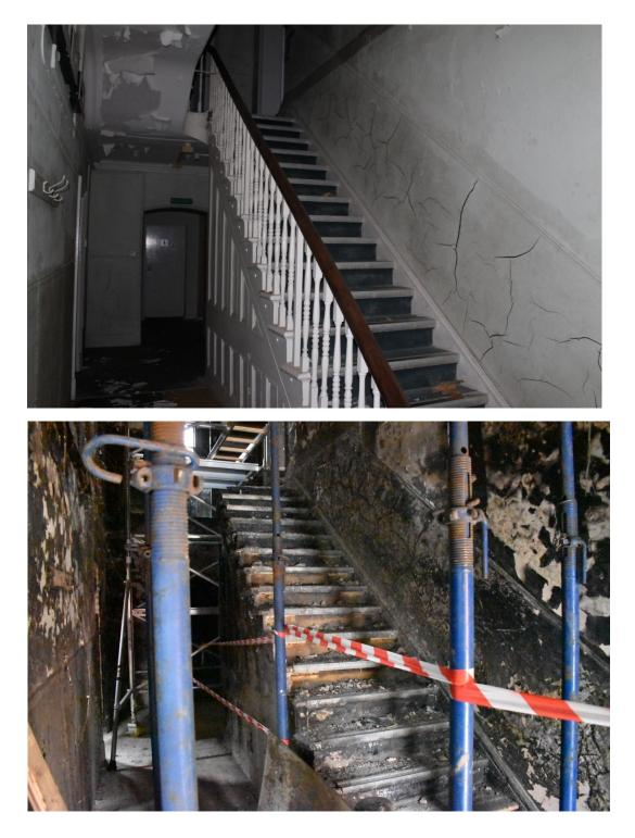
Plate 2Stairwell *iv*, showing the original staircase, coat hooks and the entrance to the<br/>1904 lavatory – view north-west. Photo from November 2013 above, photo from<br/>December 2019 below.
