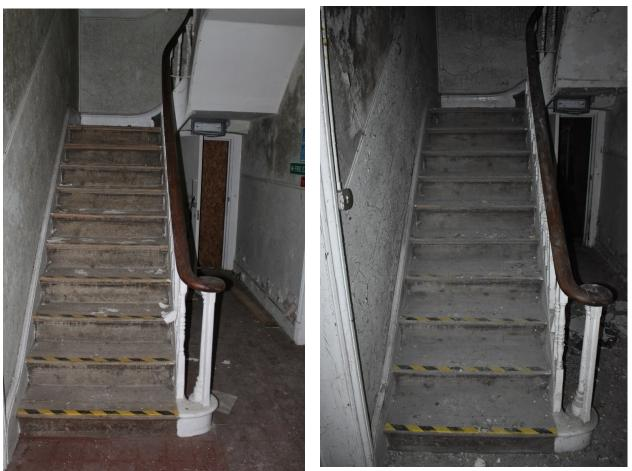
**Plate 21** Stairwell *v*, the basement stairs with the same mahogany banister with spiral end and turned balusters as the staircases of the entrance ways – view north-west. Photo from November 2013 left, photo from December 2019 right.
