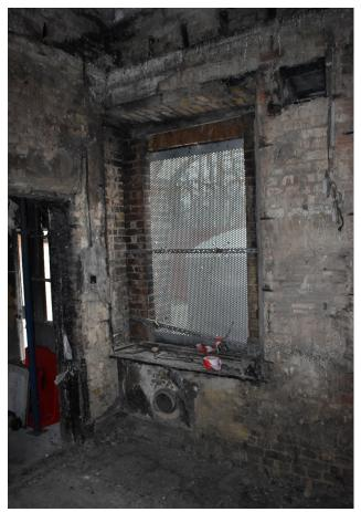
**Plate 23** Detail of window opening on ground-floor of building below room 25, showing complete destruction of window-frame by fire – view east.
