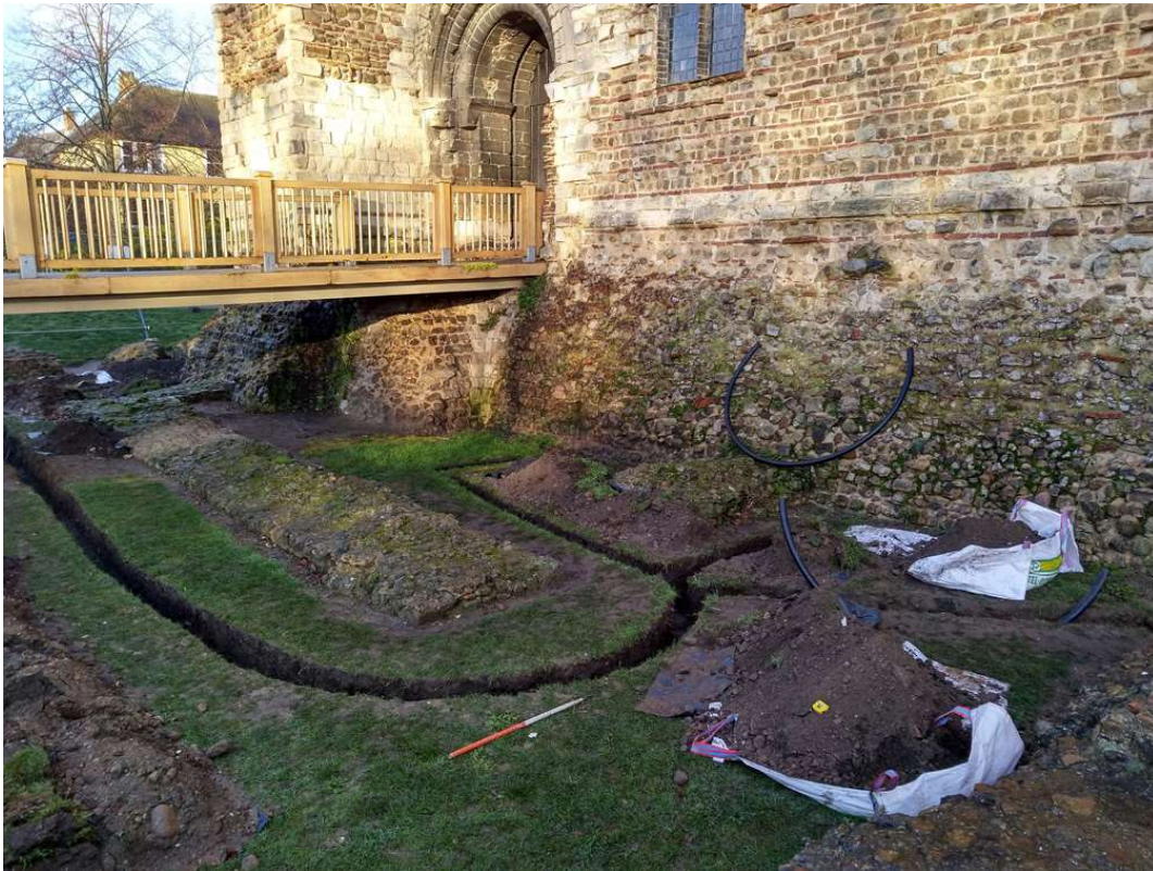
Photograph 2 New cable trench, looking northwest
