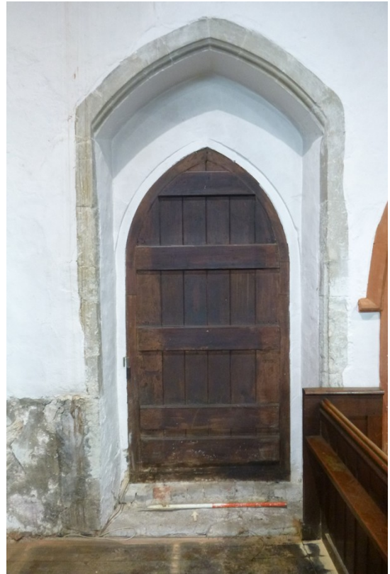
Photograph 8 Interior of doorway in north aisle. Photograph taken facing north-west.
