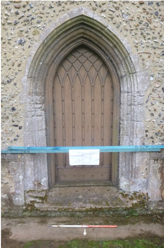
Photograph 7 Exterior of doorway in north aisle. Photograph taken facing south-east.
