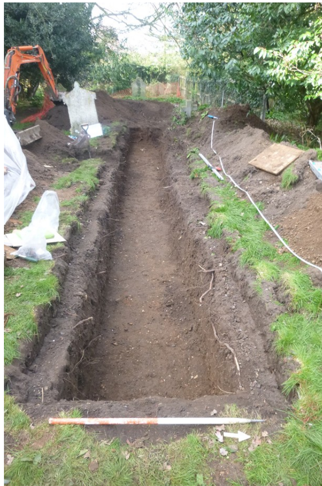
Photograph 4 Trench arch after excavation. Photograph taken facing south-west.
