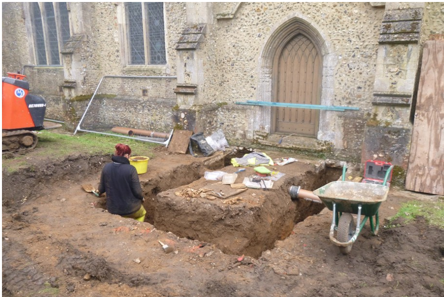
Photograph 1 Foundation trenches during monitoring. Photograph taken facing east.
