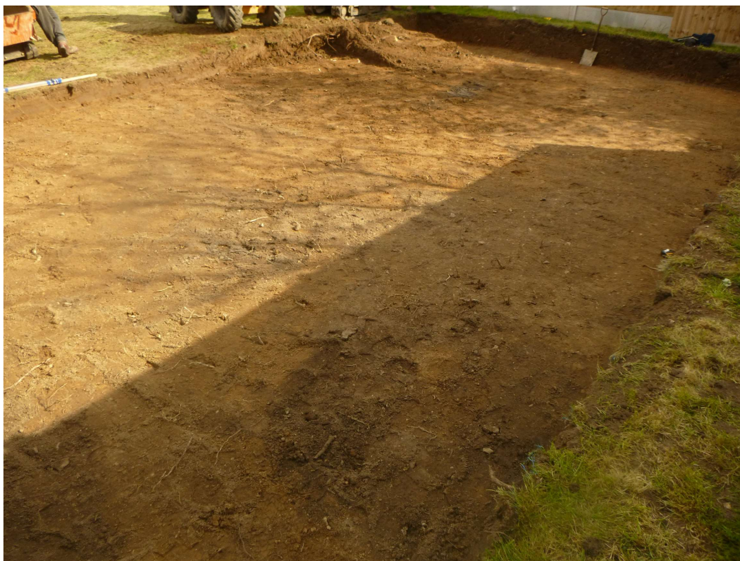
Photograph 1 The area strip for the building at the end of the garden, with F2 in the foreground, looking northwest
