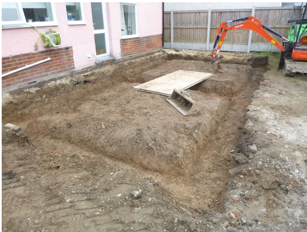
Photograph 2 The foundation trenches for the rear extension, looking southeast
