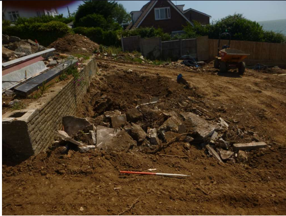
Photograph 2 Demolition of staircase – looking east
