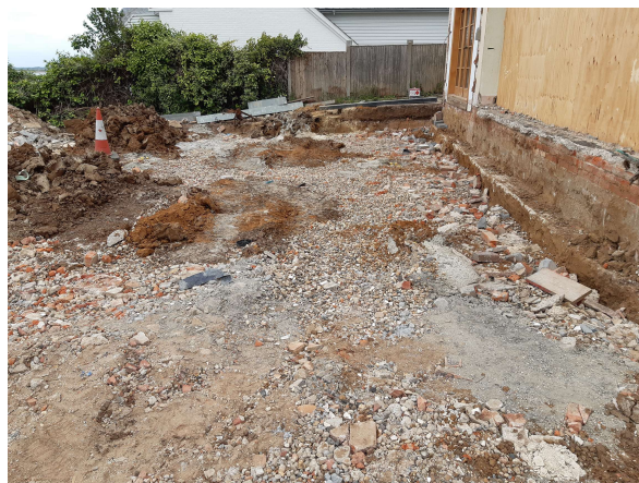
Photograph 1 Area of extension during ground reduction – looking west
