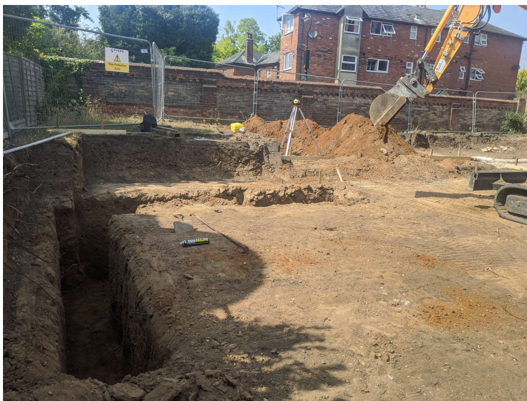
Photograph 13 Ground reduction and foundation trenches to south of site, looking west
