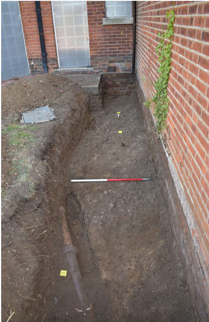
Photograph 7 The lightwell trench with metalised road surface F2, looking north
