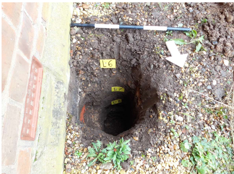
Photograph 3 FH1, looking south
