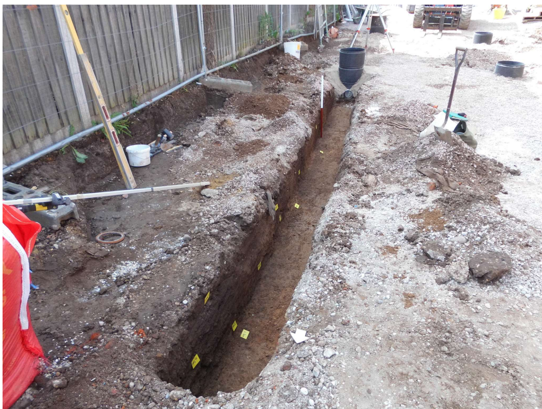
Photograph 17 Service trench 3, looking south
