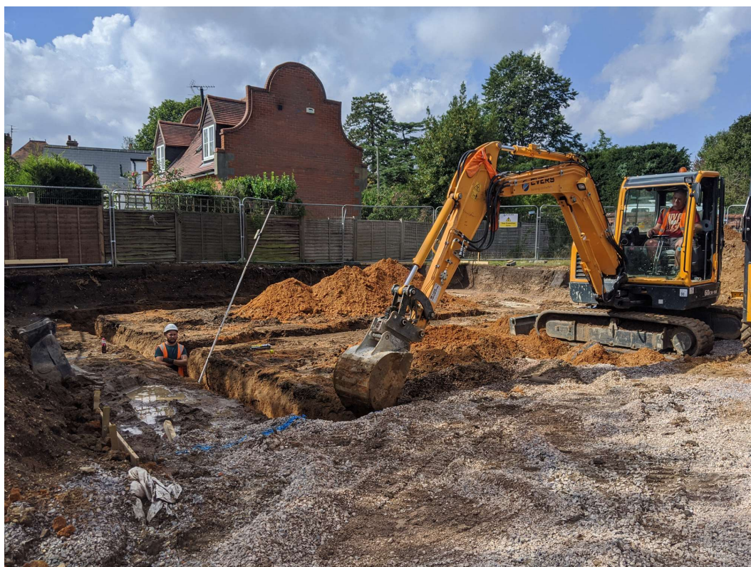
Photograph 14 Foundation trenches to south of site, looking southwest
