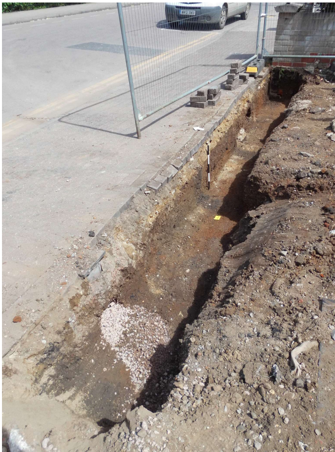
Photograph 20 Foundation trench for the new front wall, looking northeast
