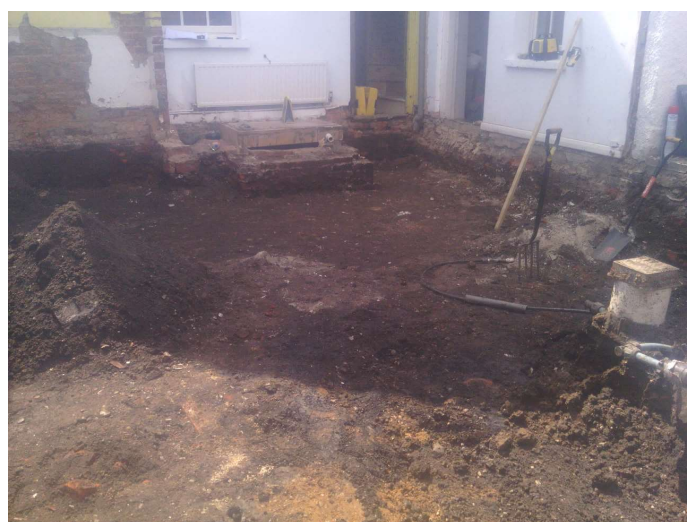
Photograph 1 Stripped area – looking south
