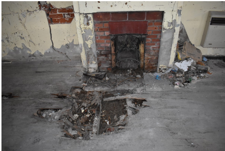
Photograph 17 Detail of inserted fireplace in western chimney-breast of southern room. Damaged section of floor visible in front. Photograph taken facing north-west.
