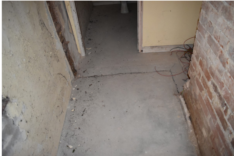
Photograph 23 Detail of scarring on floor of north room, showing location of original brick wall forming end of corridor. Location of original entrance into building to the left. Photograph taken facing north-west.
