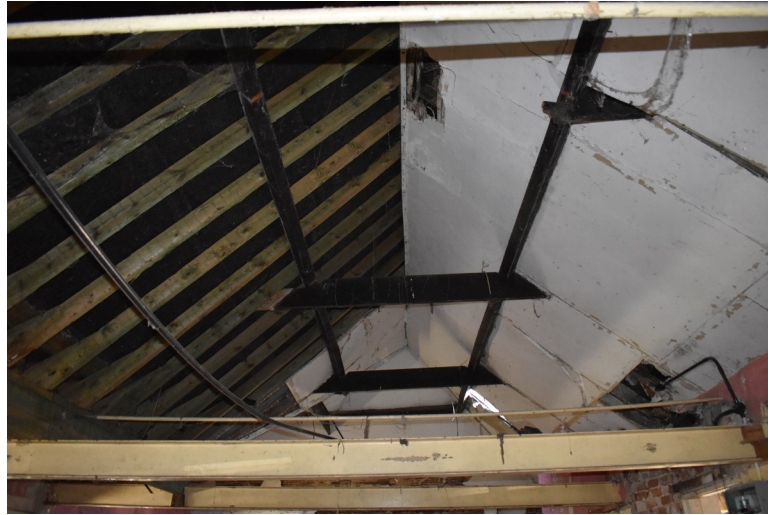
Photograph 21 Detail of roof structure above cross-wing. Rafters on left side are replacement timbers. Photograph taken facing north-west.
