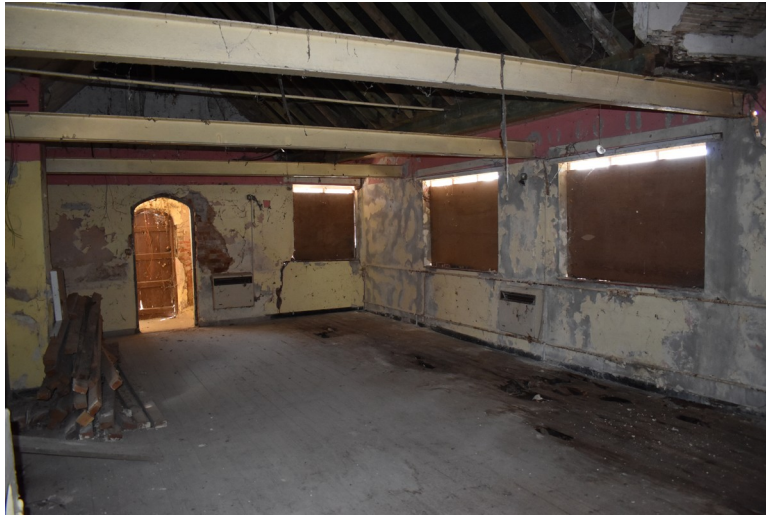
Photograph 16 Southern room of building, showing metal beams and damaged floorboards. Photograph taken facing east.
