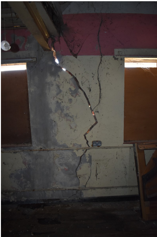
Photograph 19 Serious structural problems evident on south-east elevation of southern room. Photograph taken facing south-east.
