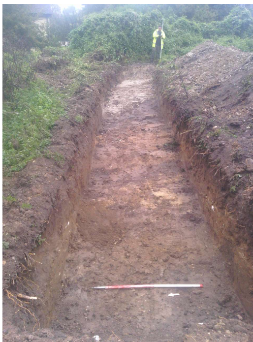
Photograph 1 T3 trench shot – looking east
