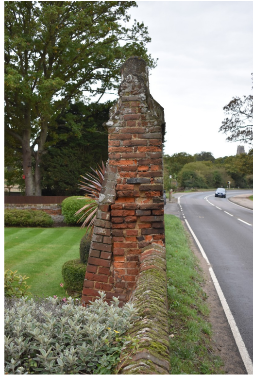
Photograph 4 North-east elevation of gateway. Photograph taken facing south-west.
