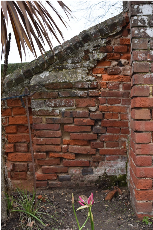
Photograph 6 Detail of section of wall immediately to south of gateway, showing 16th-century brickwork in front of later, thicker, brickwork. Also visible is significant damage in top right of frame. Photograph taken facing north-west.
