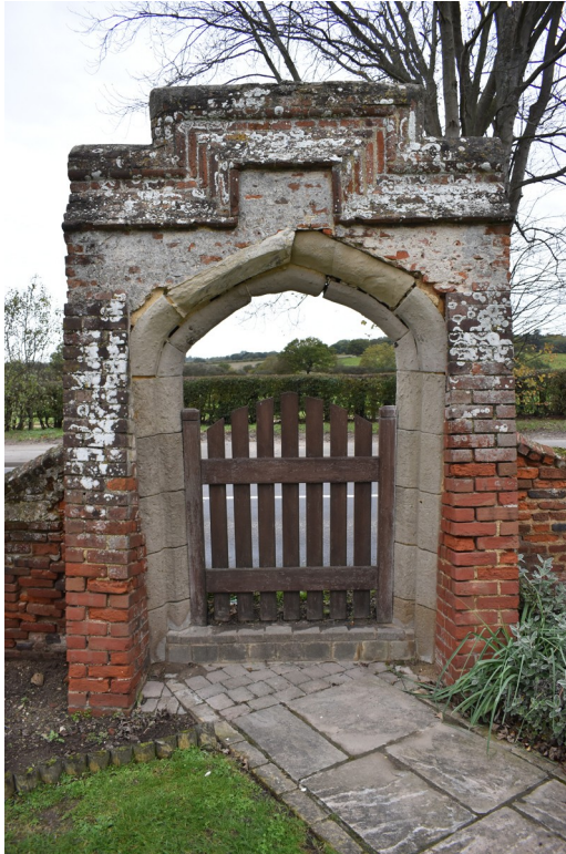
Photograph 1 South-east elevation of the gateway, showing buttresses. Photograph taken facing north-west.
