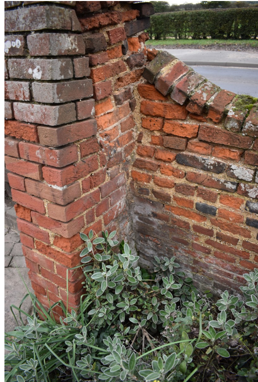
Photograph 7 Detail of north-eastern elevation of gateway, showing join with garden wall and varied brickwork. Photograph taken facing west.
