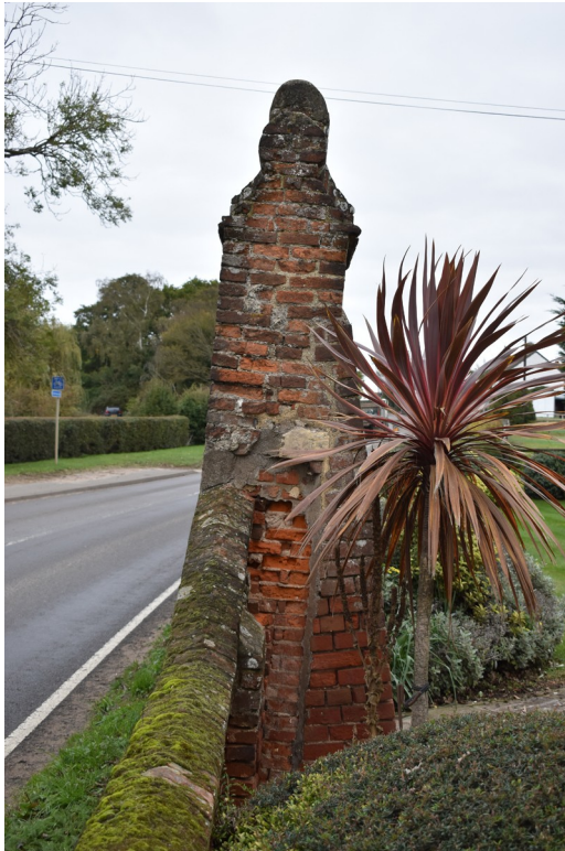
Photograph 3 South-west elevation of gateway. Damage to brickwork visible. Photograph taken facing north-east.
