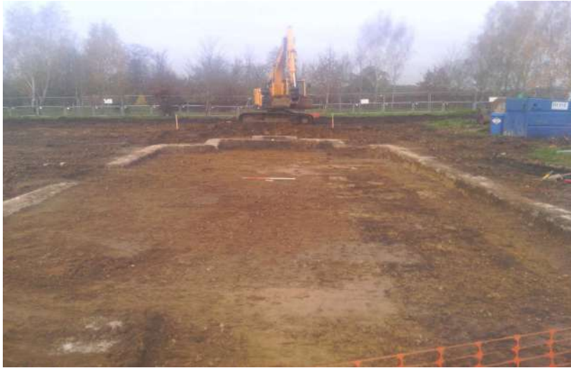
Photograph 3 Area 3 shot – looking west
