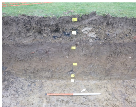
Photograph 1 Representative section of trench, showing layers. Photograph taken facing north-west.
