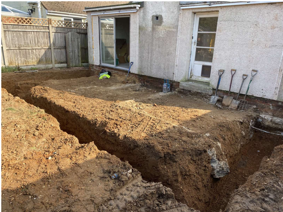
Photograph 1 The foundation trench, showing the original concrete foundations from the demolished extensions, looking east.
