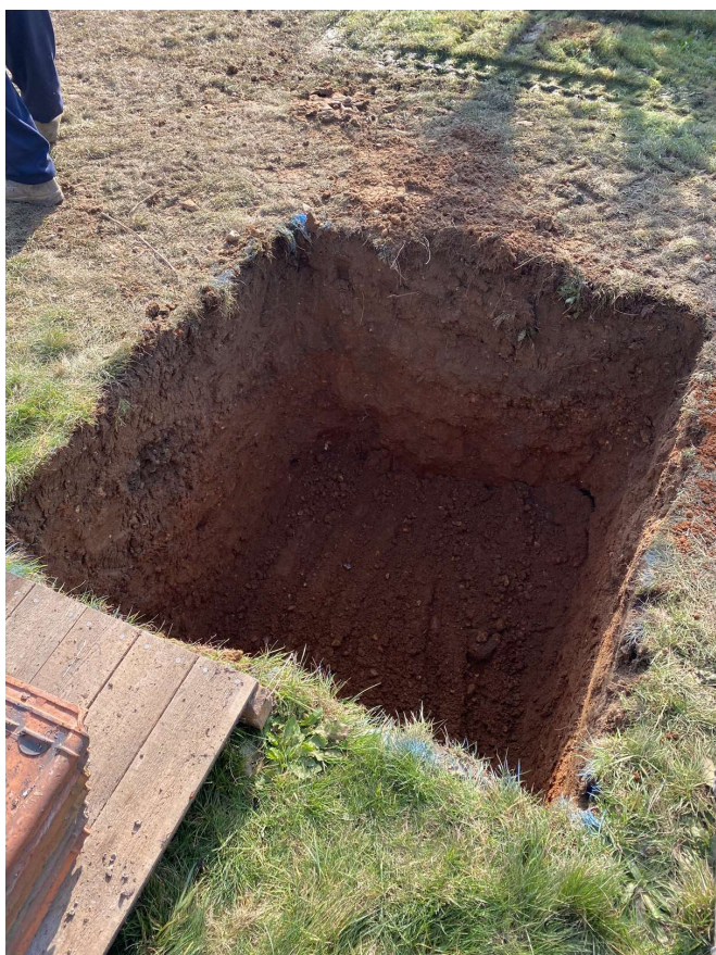
Photograph 3 The soakaway, looking west
