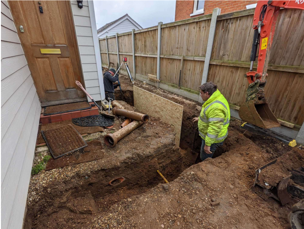
Photograph 2 Foundation trenching, looking southeast
