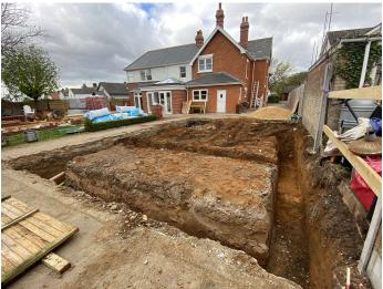
**Photograph 1** Site shot showing foundation trenching for the new garage – looking west southwest
