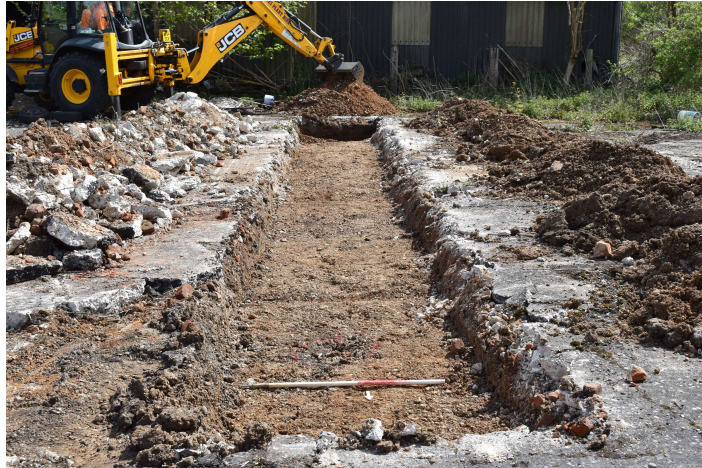
Photograph 1 T1 trench shot – looking south
