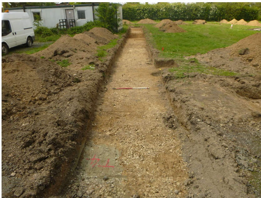
Photograph 1 T4 trench shot – looking northwest
