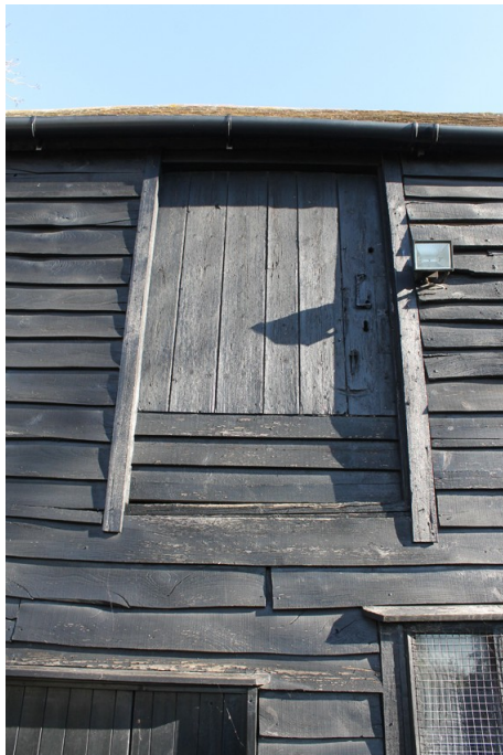
Photograph 2 Detail of pitching-door on southern elevation. Photograph taken facing north.
