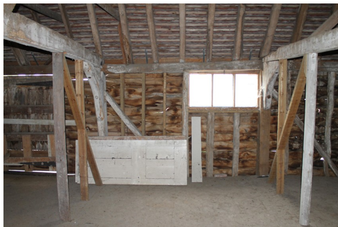
Photograph 17 Southern elevation of bay 2 on first-floor, showing modern studs, window and scarf joint. Photograph taken facing south.
