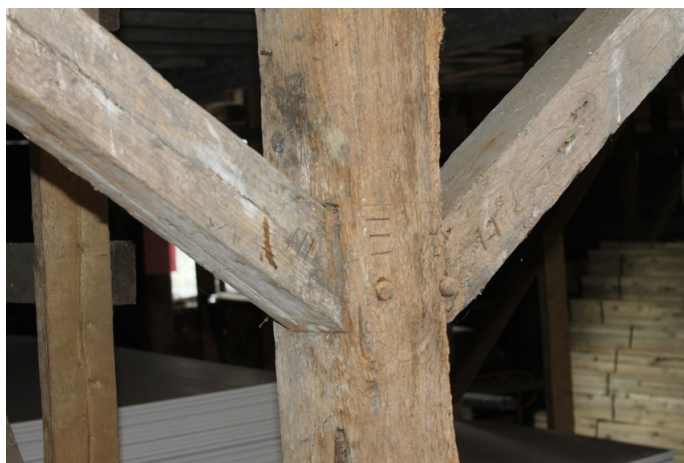
Photograph 27 Detail of northern principal-post between bays 4 and 5, showing carpenter's marks 'II' and 'III'. Photograph taken facing south-west.
