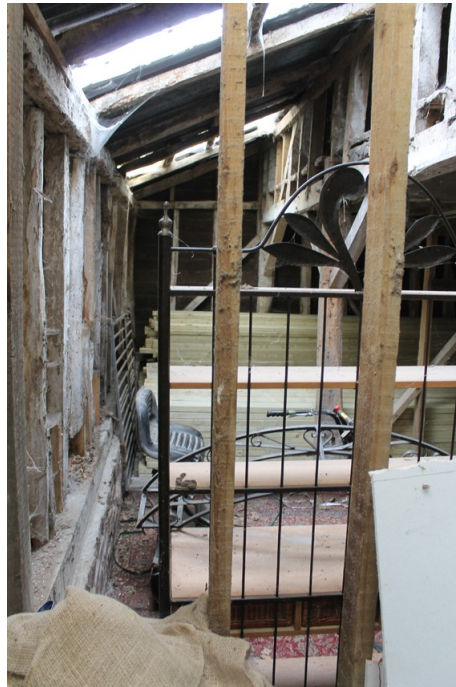
Photograph 30 Interior of lean-to, with re-used hand-sawn studs to left of frame. Photograph taken facing east.
