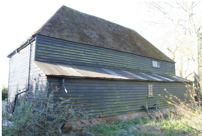
Photograph 4 Northern elevation of building, show lean-to supported on brick plinth. Photograph taken facing south-west.
