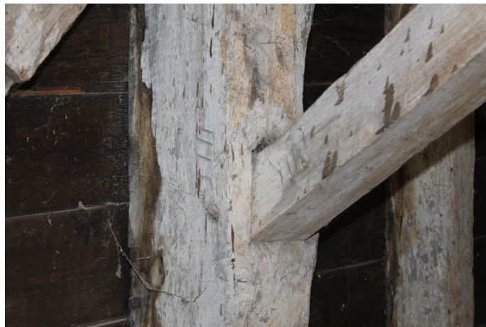
Photograph 29 Detail of north-east corner-post of building, showing carpenter's mark 'IIII' on post and brace. Photograph taken facing south-east.
