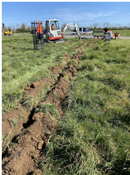
Photograph 1 Cable trenching – looking northeast
