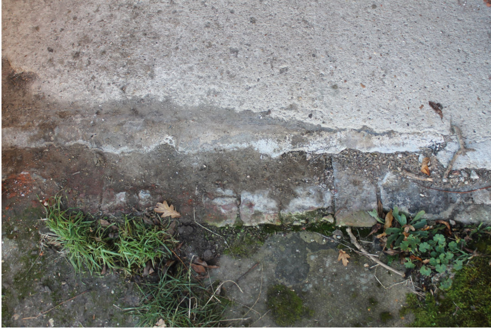
Photograph 13 Detail of original brick flooring covered with concrete. Photograph taken facing south-east.
