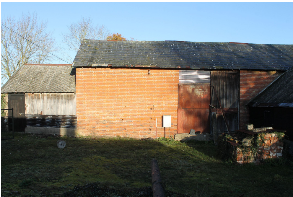
Photograph 3 South-eastern elevation. Photograph taken facing north-west.
