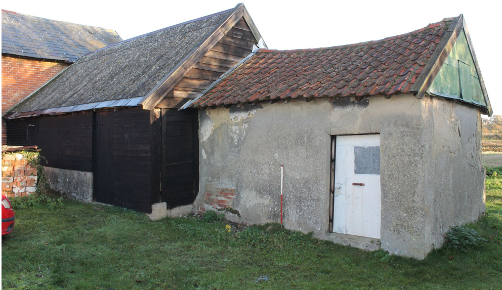
Photograph 10 South-western elevation of outbuilding 5. Photograph taken facing north.
