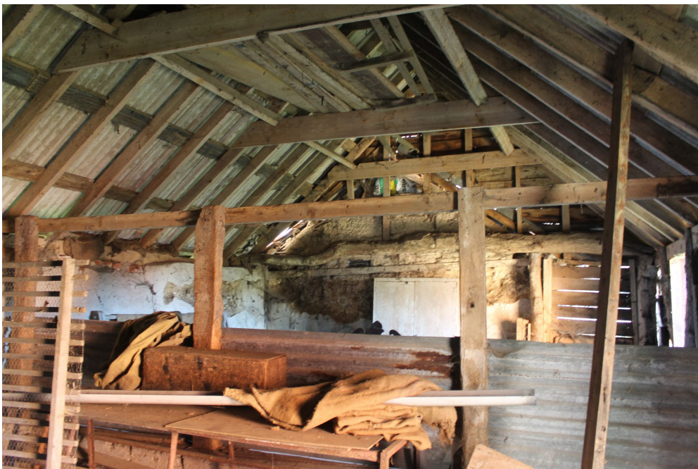
Photograph 17 Interior of outbuilding 4. Photograph taken facing south-east.
