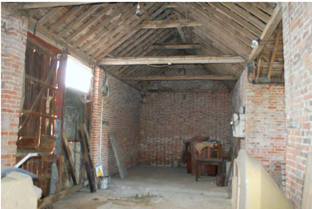
Photograph 12 Interior of threshing barn. Photograph taken facing south-west.
