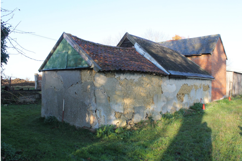
Photograph 9 Detail of clay wall on north-eastern and south-eastern elevations. Photograph taken facing north-west.
