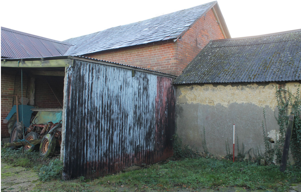
Photograph 2 North-western elevation. Photograph taken facing east.
