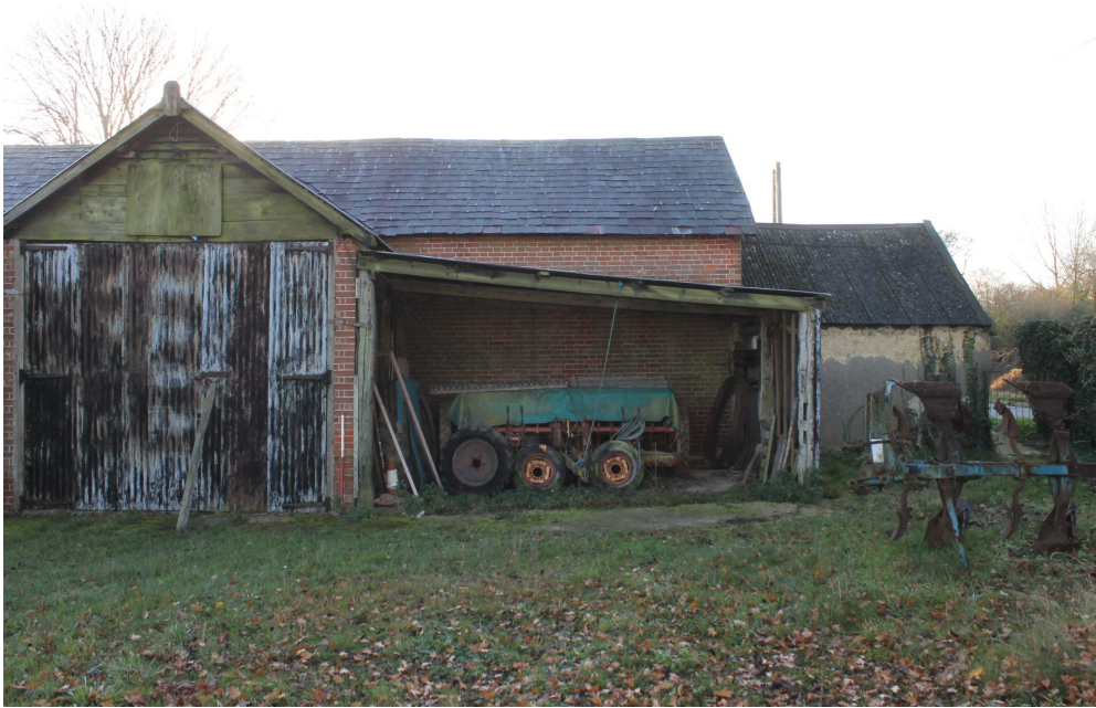
Photograph 8 Outbuilding 2 on north-western elevation. Photograph taken facing south-east.
