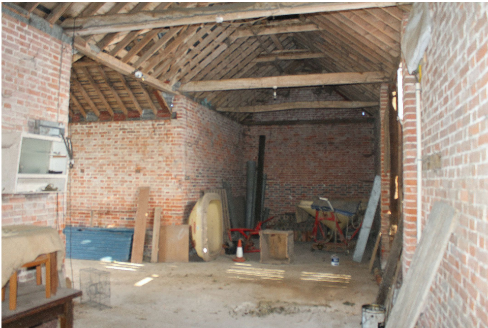
Photograph 11 Interior of threshing barn. Photograph taken facing north-east.
