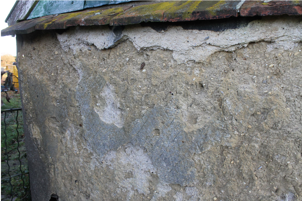
Photograph 6 Detail of surviving keyed horsehair plaster on clay wall of western elevation. Photograph taken facing north-east.
