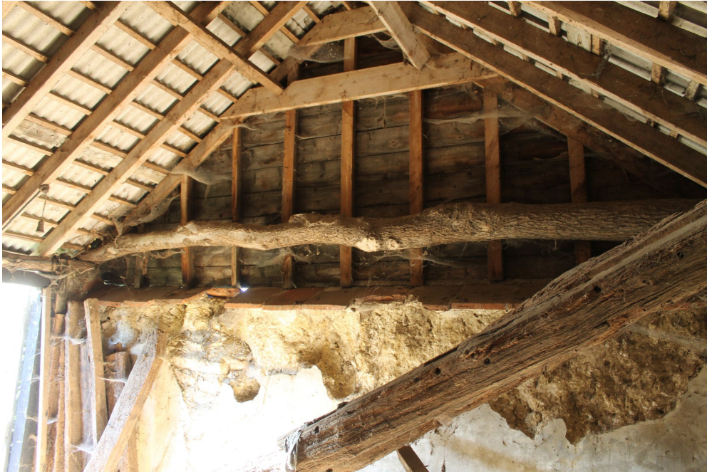
Photograph 16 Interior of outbuilding 1 showing detail of timber structure. Photograph taken facing south-west.
