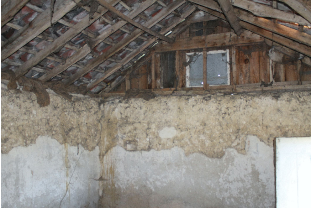
Photograph 18 Interior of outbuilding 5. Photograph taken facing south-east.
