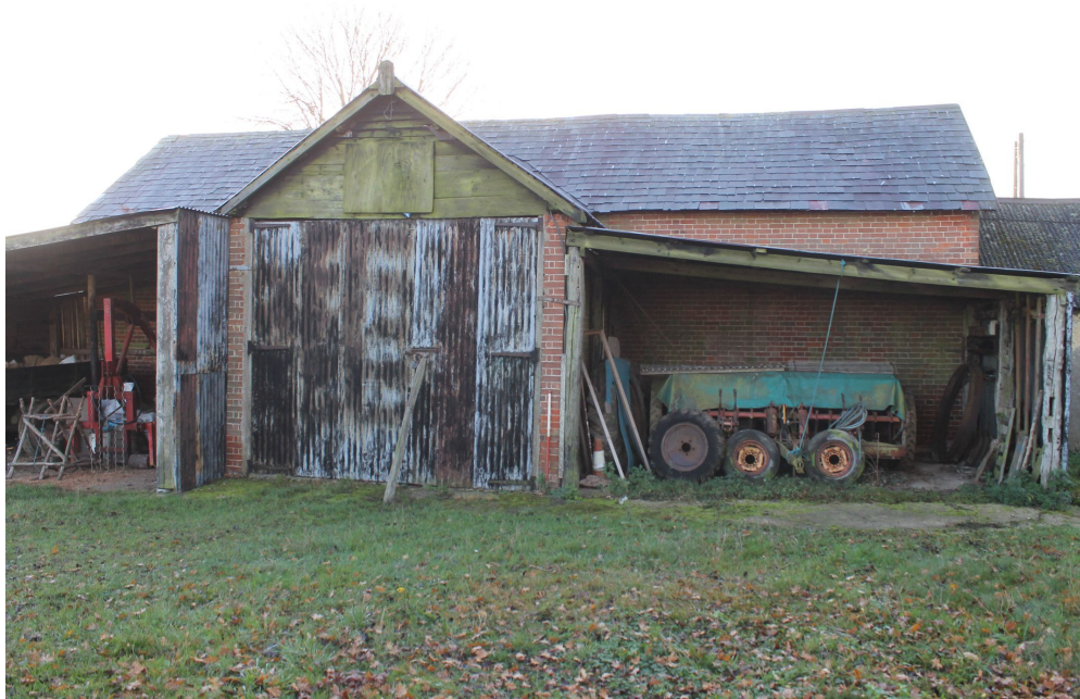
Photograph 1 North-western elevation. Photograph taken facing south-east.
