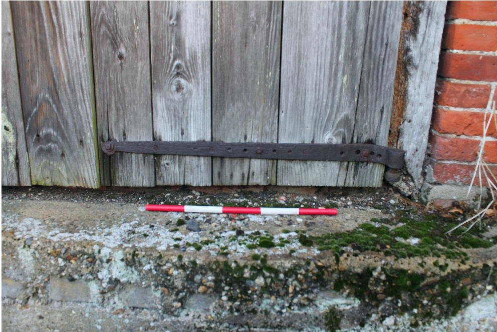
Photograph 4 Detail of original hinge and pintles. Photograph taken facing north-west.
