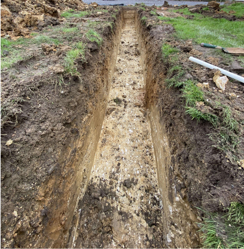
Photograph 3 NW-SE trench on the north side of site, looking roughly north-west.
