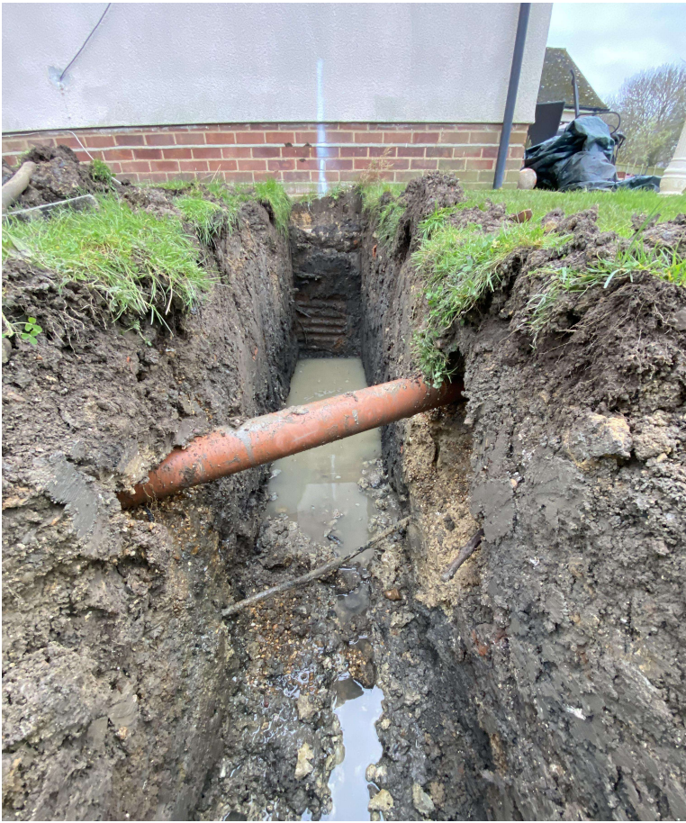
Photograph 4 Trench on the south-west of site, showing modern services and flooding from water pipe, looking south-east.
