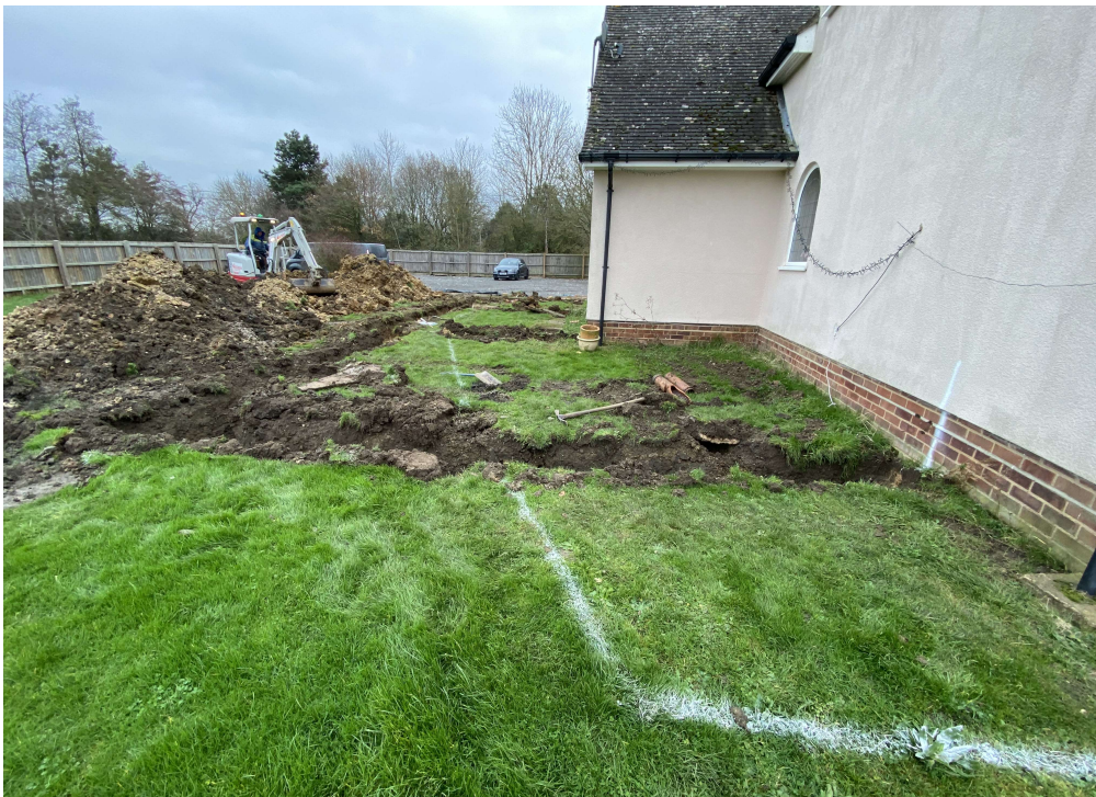
Photograph 2 Trenches from west end of site, looking north-east.
