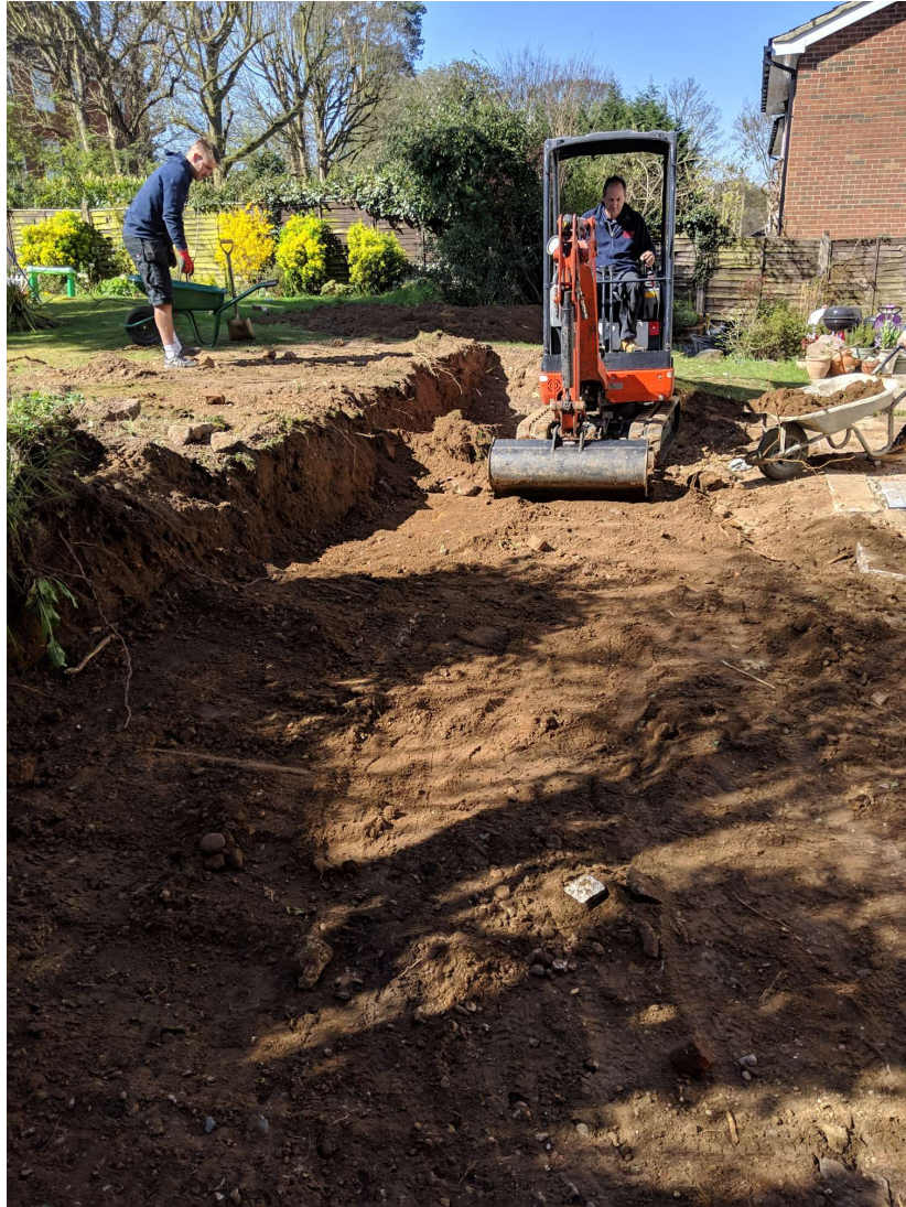
Photograph 2 Working shot - view west
