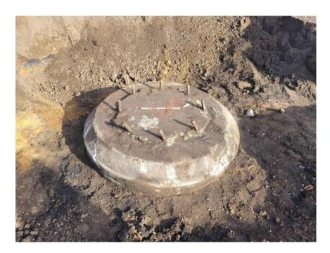
Photograph 1 Central pivot of the turntable, looking north-west
