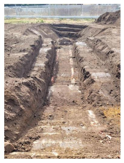
Photograph 2 Looking down into turntable pit, showing staircase, external concrete ring, brick walls and central pivot, looking south-west
