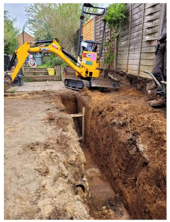
**Photograph 2** Foundation trenching looking north-west
