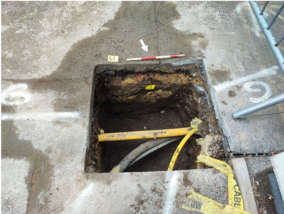
Photograph 2 Pad 6, looking south-west
