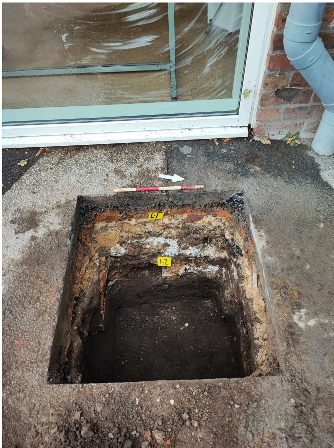
Photograph 3 Pad 9, looking east
