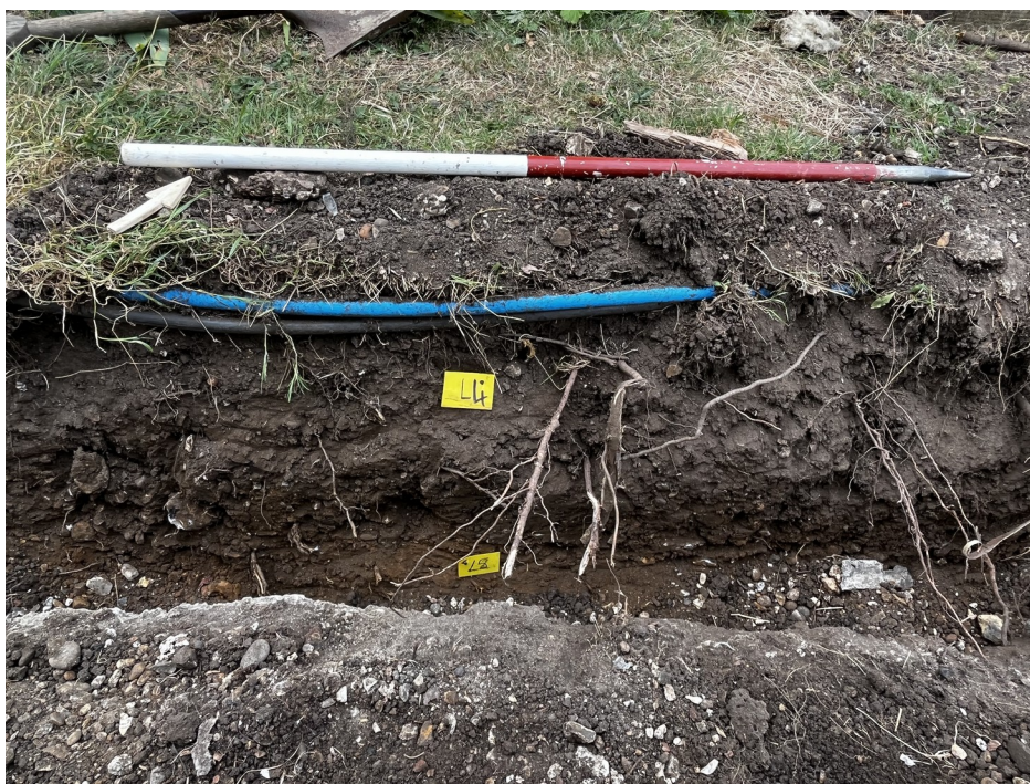
Photograph 4 Section of footings showing modern pipes and significant rooting. Looking roughly north-west.
