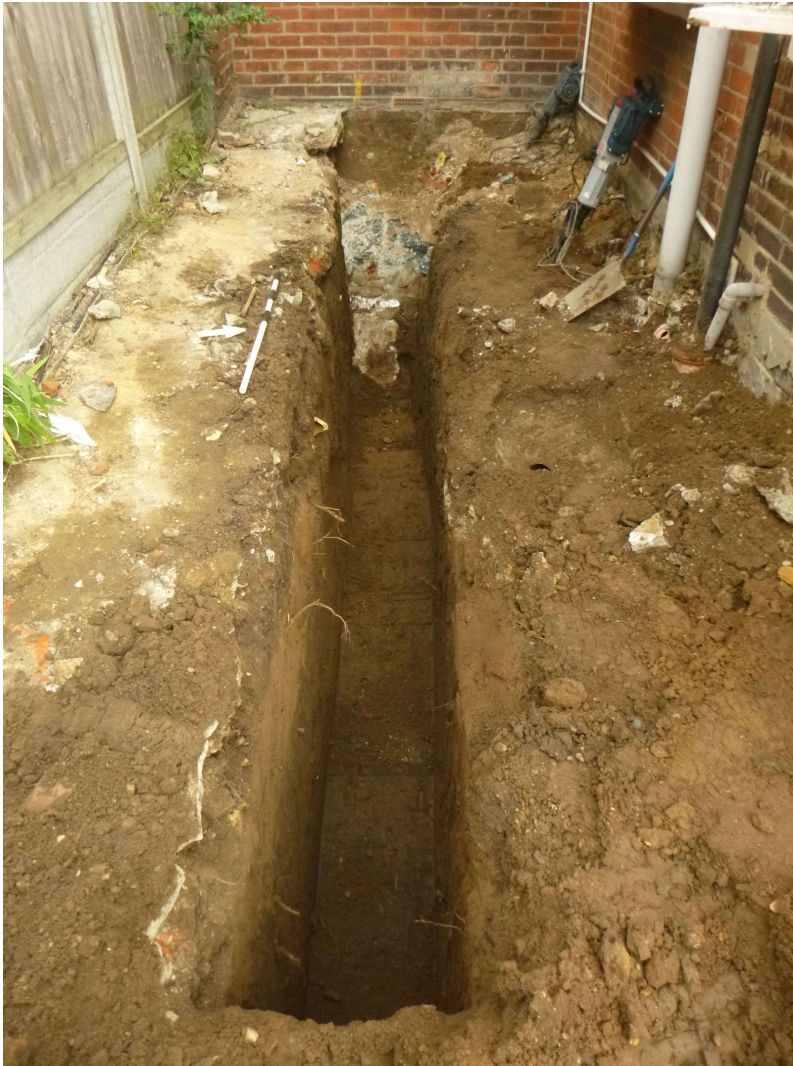
Photograph 1 Foundation trench, looking north
