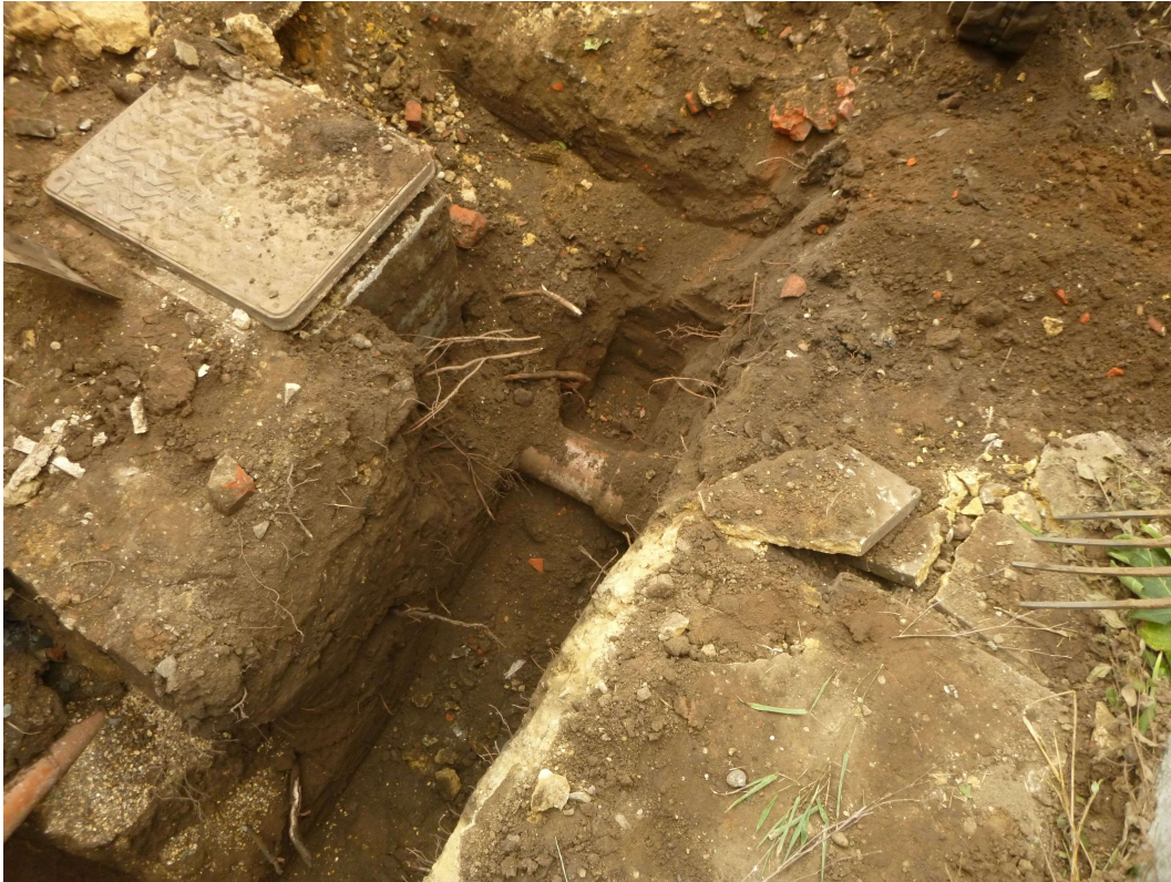
Photograph 2 South-west corner of foundation trench showing manhole and services, looking south
