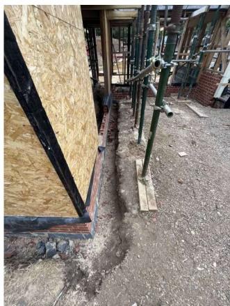
**Photograph 8** One of the underpinning trenches around the centre of the outbuilding, looking east-south-east
