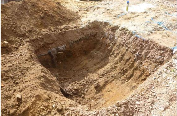
Photograph 18 Working shot of septic tank excavation
