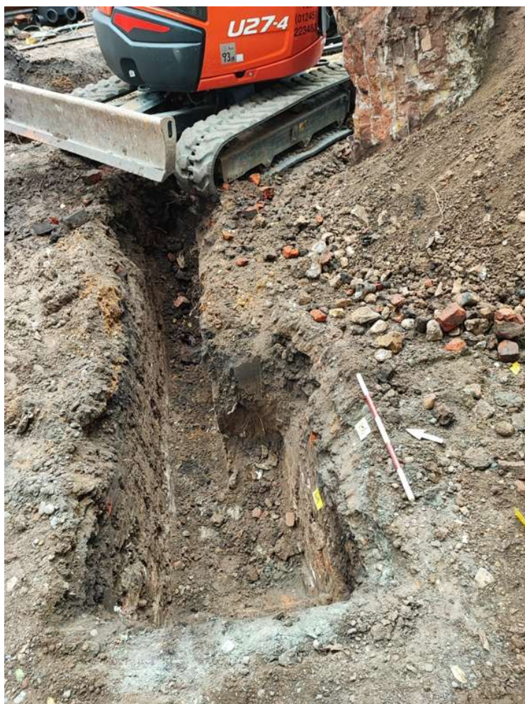
Photograph 3 Manhole and drainage trench – view east.
