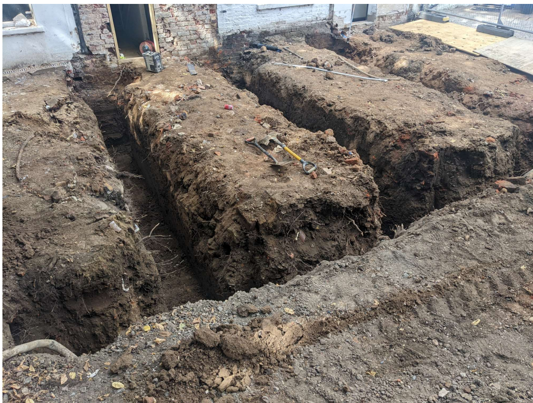
Photograph 1 Foundation trenches – view north.
