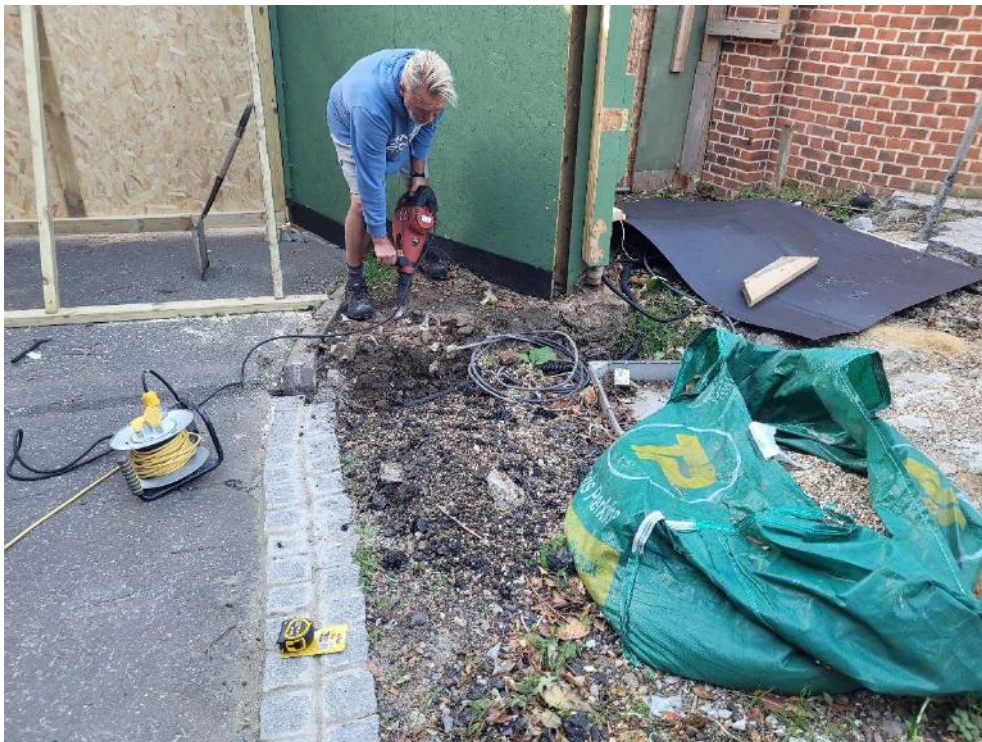
Photograph 1 Working shot of first foundation pad being excavated, looking west
