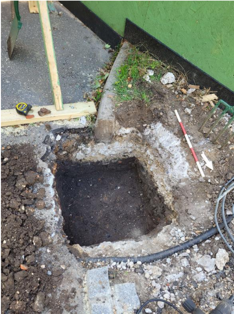
Photograph 2 Post-excitation shot of foundation pad 1, looking south-south-west
