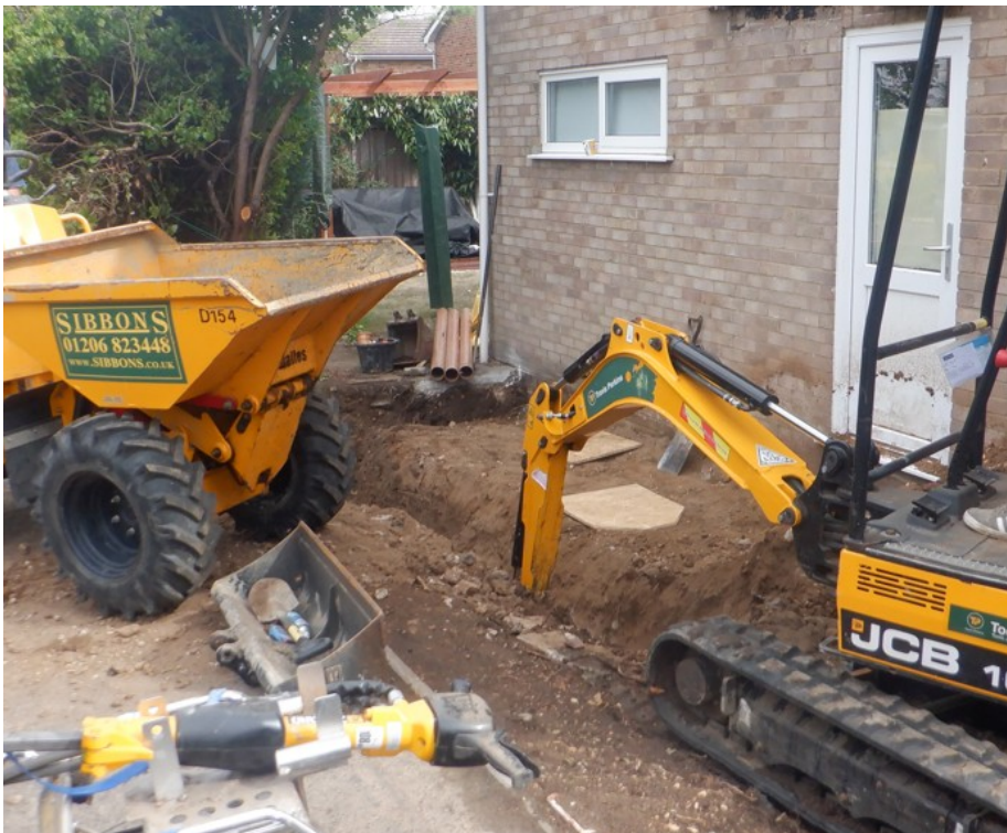
Photograph 2 General view of foundation trench excavations, looking north-east
