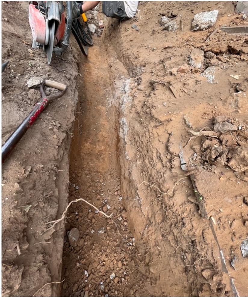
Photograph 3 General view of foundation trench south-west corner, looking north
