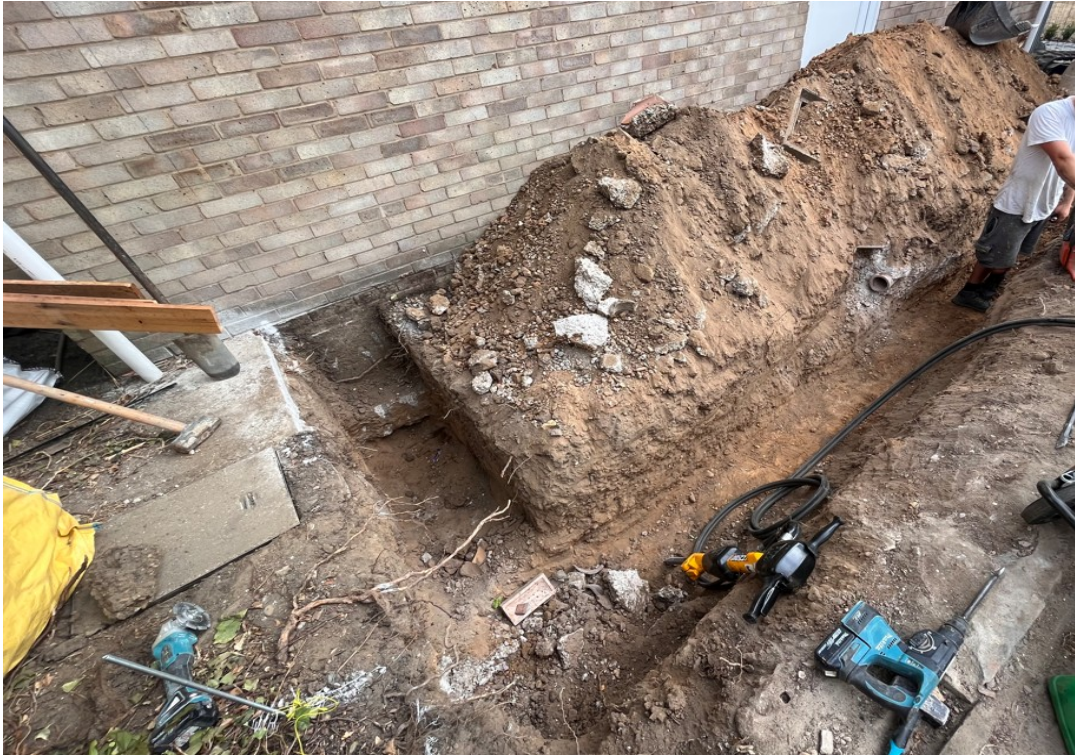
Photograph 1 General view of foundation trench in north-west corner, looking south-east
